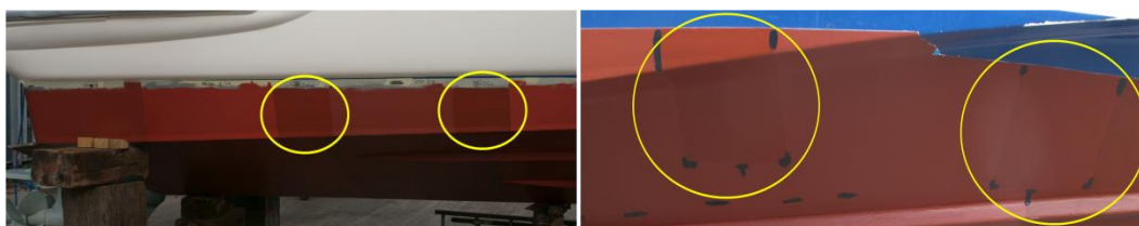
Figure 4:29: Photographs of the stern (right) and bow (left) starboard sections of the test patching vessel. Yellow circles indicate AMPSQ coating test patches
