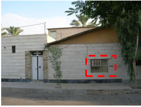
Fig. 14 An instance for the applied electrical active air-conditioning system in Lar
