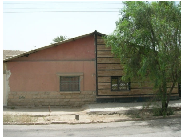
Fig. 8 Twin prefabricated houses in New Lar city
