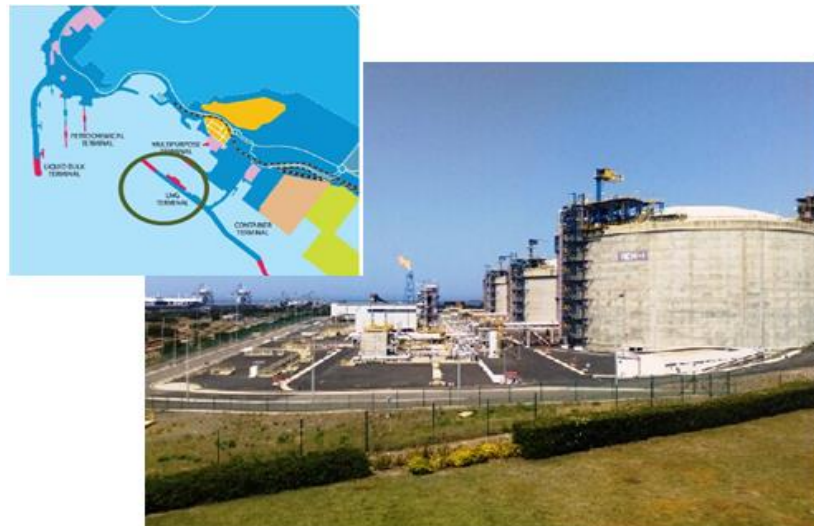
Figure A-1: Sines LNG terminal, storage tanks and terminal location.
