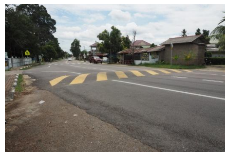
Figure 8 - Road Safety Measures or School Zone
