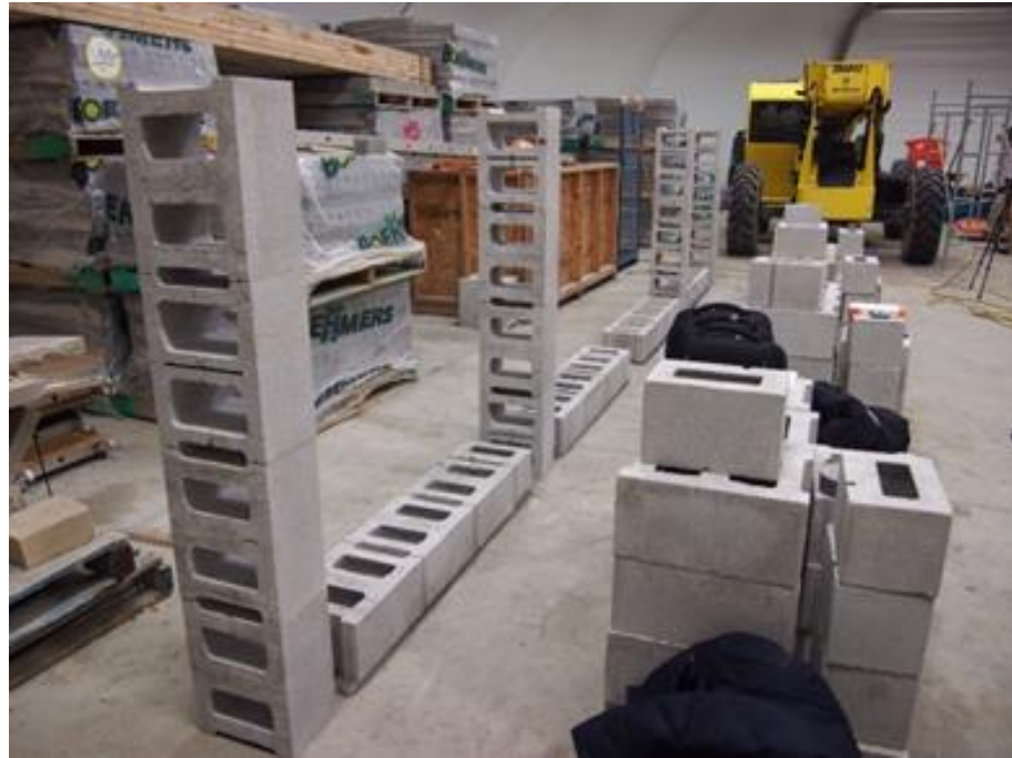
Figure 18 Experimental setup for bricklaying task
