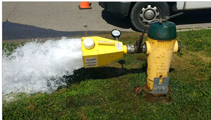
Figure 4.19: Water flowing from a hydrant port valve during field tests.
