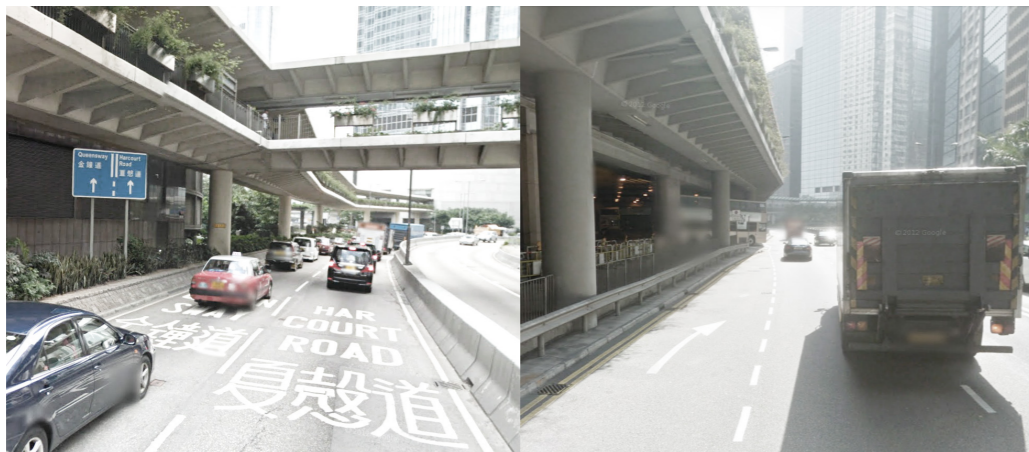
1. the absent of traffic light allows the vehicle move in high speed and the cyclists need to compete with the vehicles. 2. the present of sidewalk railing and narrow roadside increase the danger on the cyclists.
