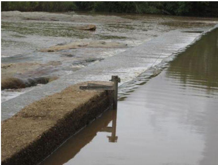
Figure D2 An illustration of the Solinst Level Logger installed at the Mahale weir to record streamflow head, which was installed on 22 April 2015 (Riddell et al., 2017)
