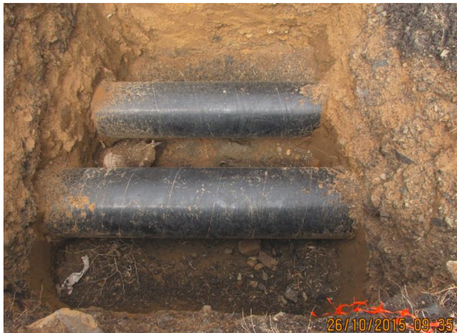
Figure-2.3 Verification dig to confirm DCVG result of good pipe coating.
