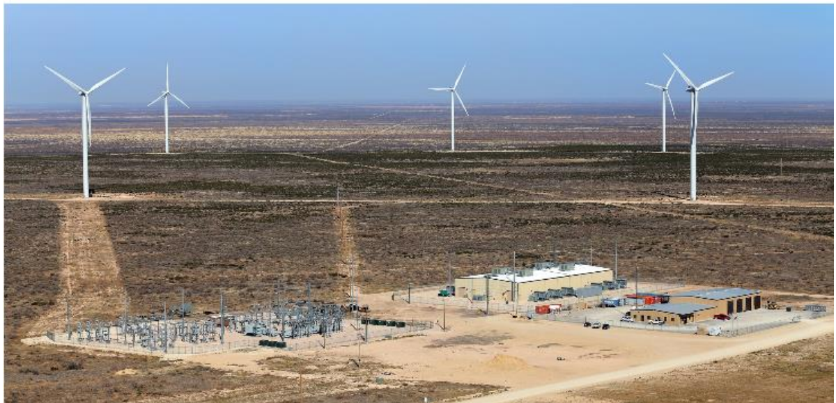
Figure 18: 36 MW Battery Storage for 153 MW Wind Integration, Source: Duke Energy, Texas
