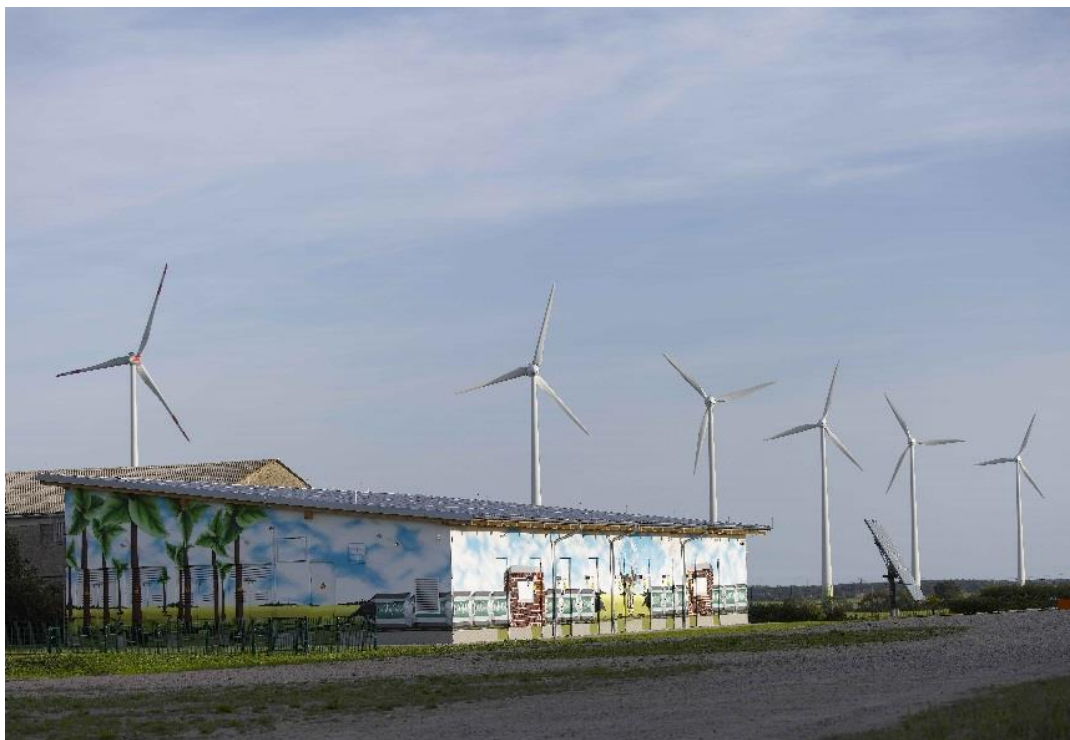
Figure 38: Brandenburg, Germany. 10MW lithium ion battery system [45]
