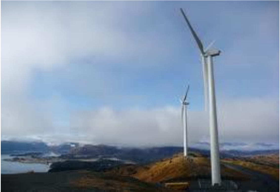
Figure 25: Kodiak Island, Alaska, 3MW advanced lead acid battery system [45]
