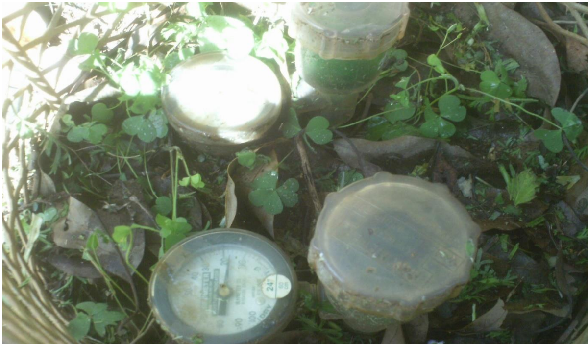
Figure 3.3 Tensiometers installed adjacent to each other at 300 and 600 mm soil depths
