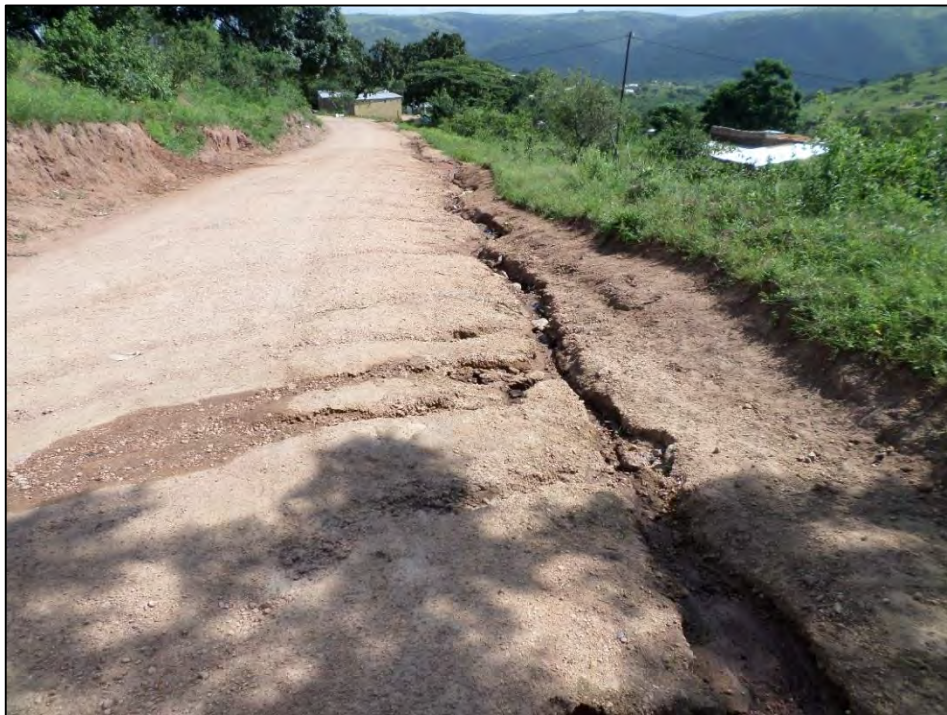
Image 5.7: Condition of some of the Roads
