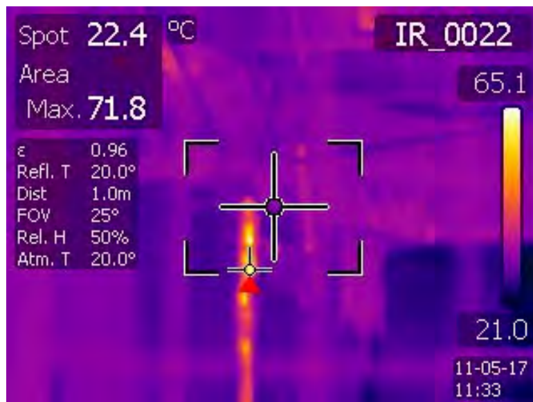
Figure 4.2 Thermal scan on 150 cm grass under the HVDC test line
