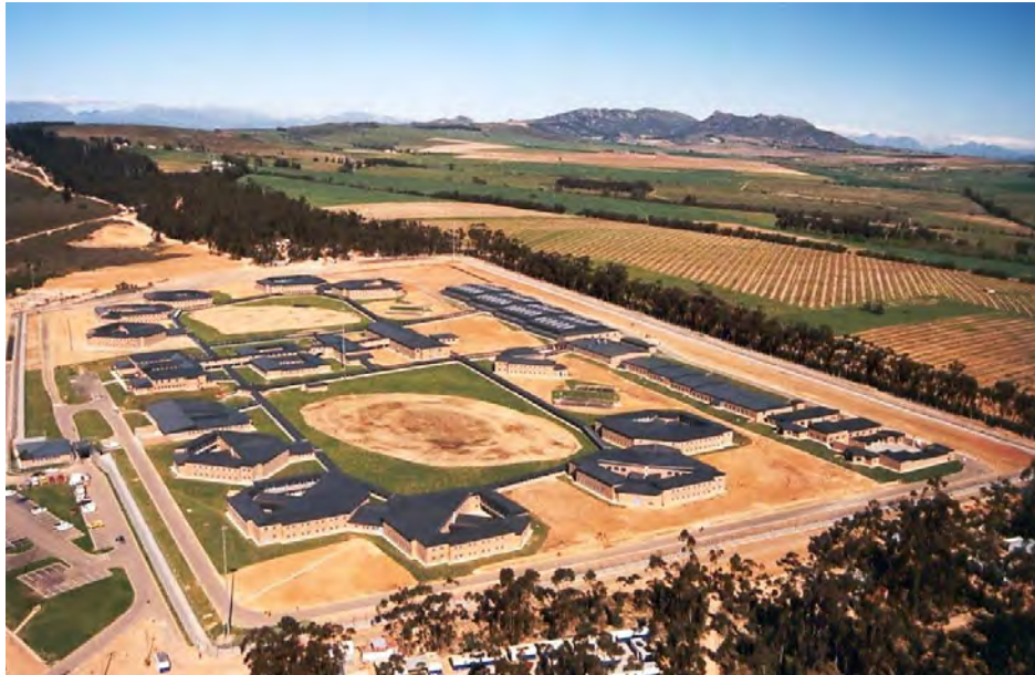
Figure 44 (Qunu Consulting (Pty) Ltd , 2009) aerial view of Malmesbury Correctional Centre showing living pods and ordered design
