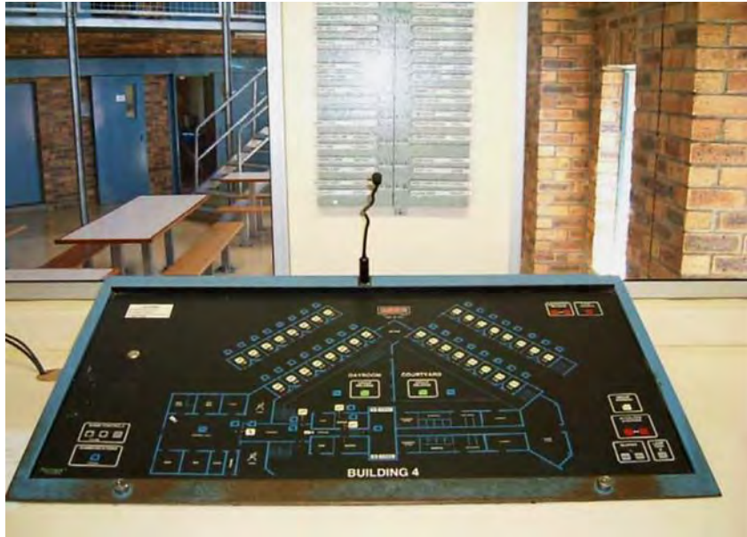
Figure 47 (Gillespie, 2010) Inside control room in cell unit/'pod', looking out onto the dayroom with cells in background
