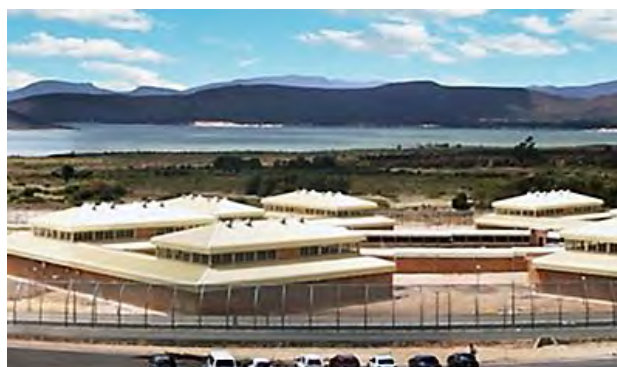
Figure 12 (eNCA, 2013) showing offenders housing facility with high security perimeter fencing
