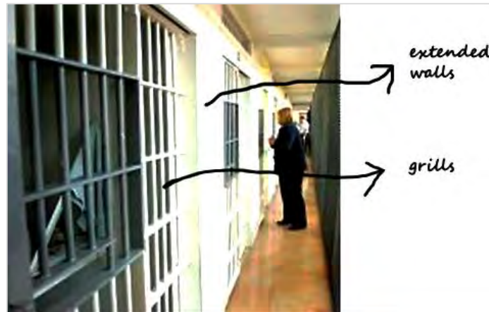
Figure 6 (Lindberg, 2013) showing Stillwater Prison built from 1910 to 1914. Grills to entrances of cells and extended walls between cells are noticeable.
