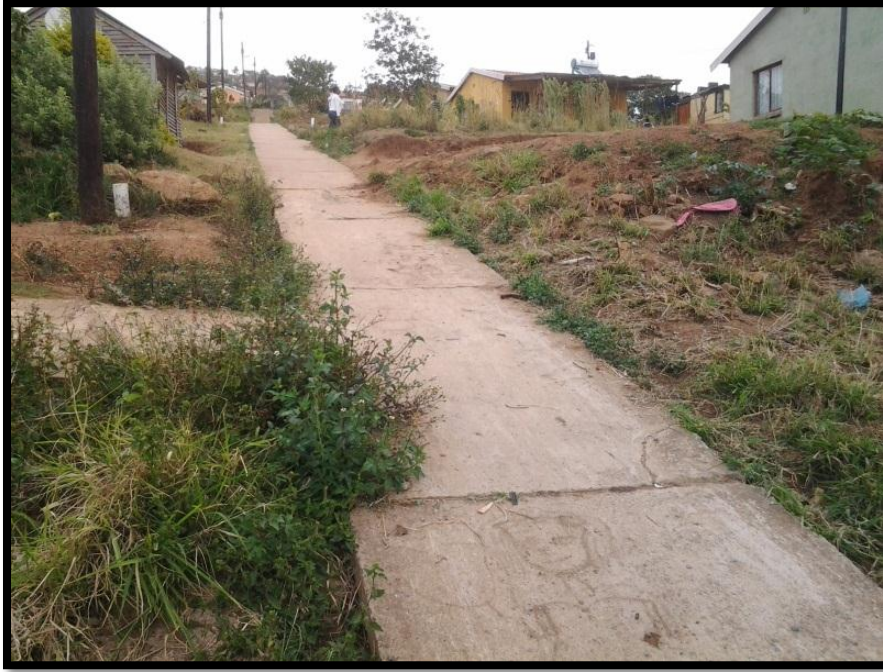
Plate 6.5: Ramps which have been built to improve accessibility
