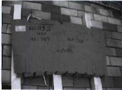
Figure 2-9: Stator core lamination plates (DTEC)
