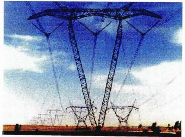
Figure 9. Guyed V Tower (765 kV)
