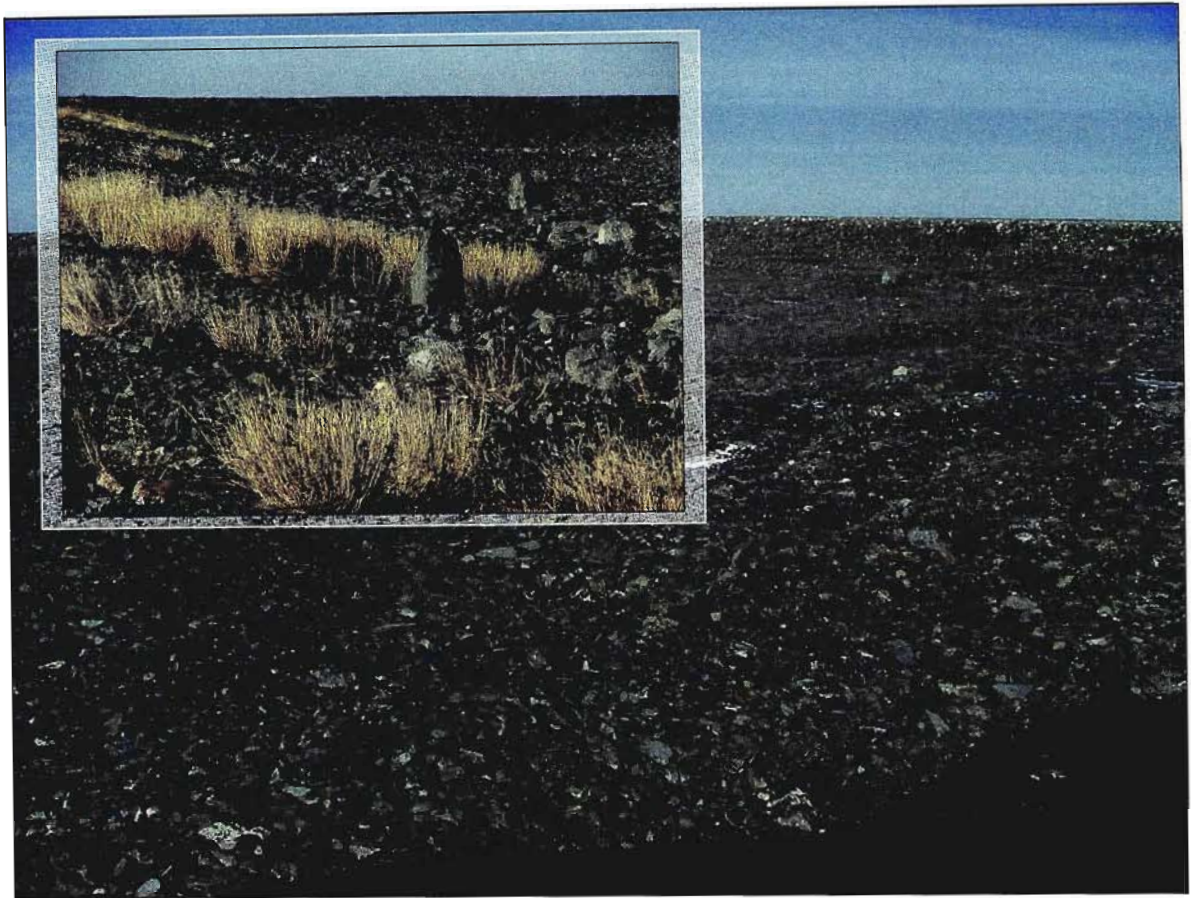
Figure 5.1 Rock cladding on the surface of the Pering Mine tailings impoundment and (inset) a view of the retainer walls.
