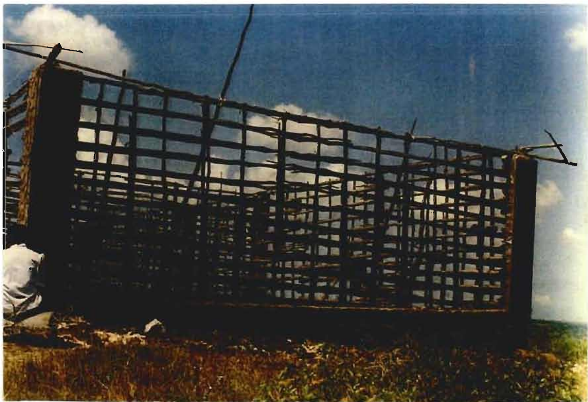
Plate 6.3: Earth-walled, angular-framed house-type, strengthened by partially cementing the walls (Photo taken in June 1999)
