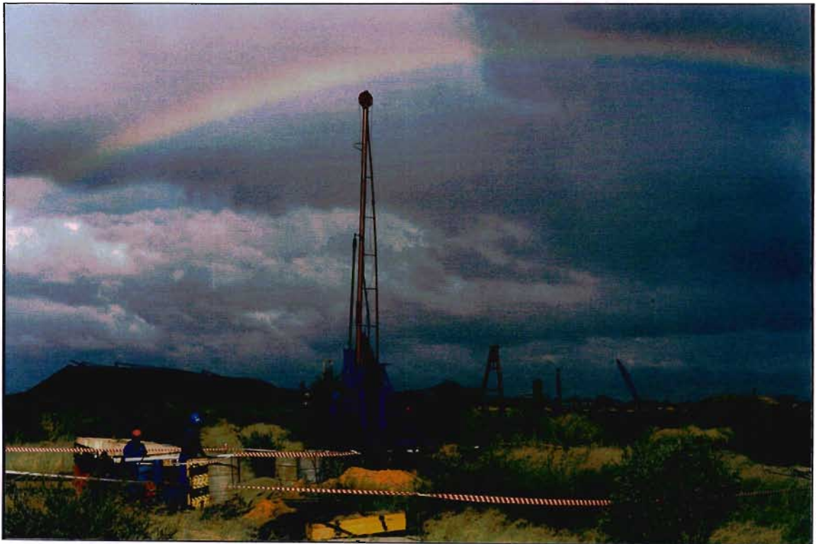
Figure 1.4 View southeast of rotary core borehole drilling ahead of the No.3 Decline Shaft development (Note the box-cut position near the orange spoil heap). (Photograph: R. Puchner, March 2000)
