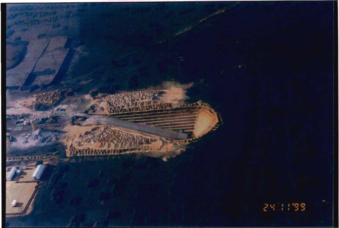
Figure 1.3 Aerial photograph showing a southward view of the Nchwaning No.3 Decline Shaft box-cut. (Photograph: C. McKnight, November 1999)
