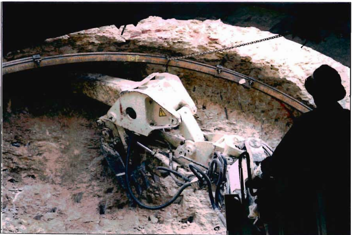
Figure 4.9 The ITC machine as it begins the tunnelling into the weathered Kalahari Group calc-arenite. (Photograph: R. Puchner, April 2000)
