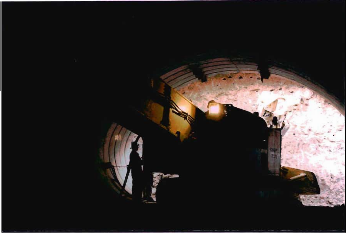
Figure 4.8 View westwards down the No.3 Decline Shaft with the ITC machine and its conveyor belt 'tail'. (Photograph: R. Puchner, April 2000)
