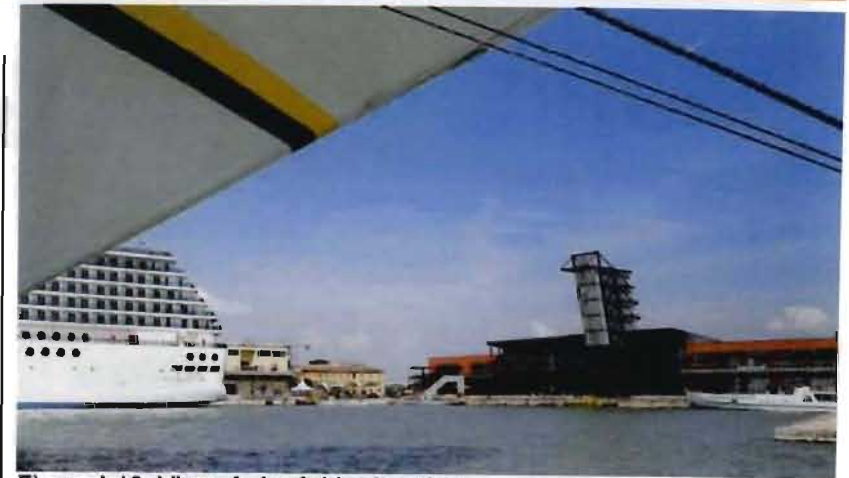
Figure 4.18 View of wharf side elevation. (Dalco. 2003: 24)
