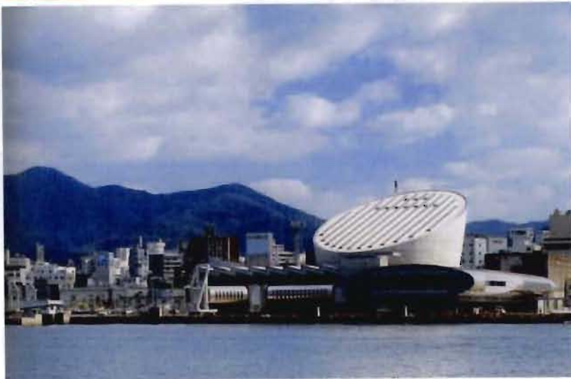
Figure 3.6_ Exterior view of Nagasaki Port Terminal. (Teramatsu. 1996: 135)
