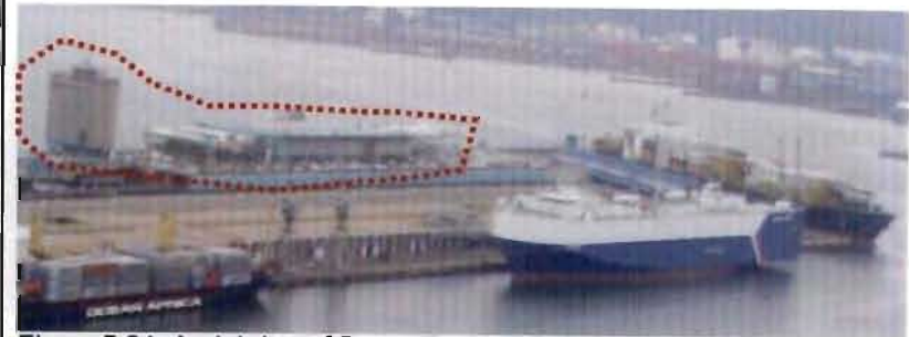
Figure 5.24_Aerial view of Ocean Terminal Building complex.
