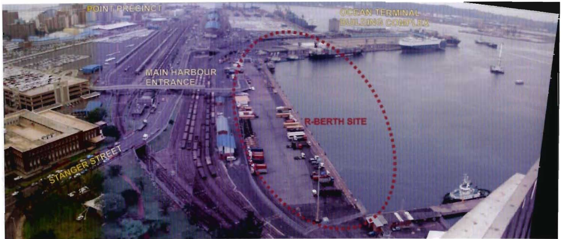
Figure 7.5_Aerial photograph of R-Berth site showing its position in relation to the main harbour entrance.
