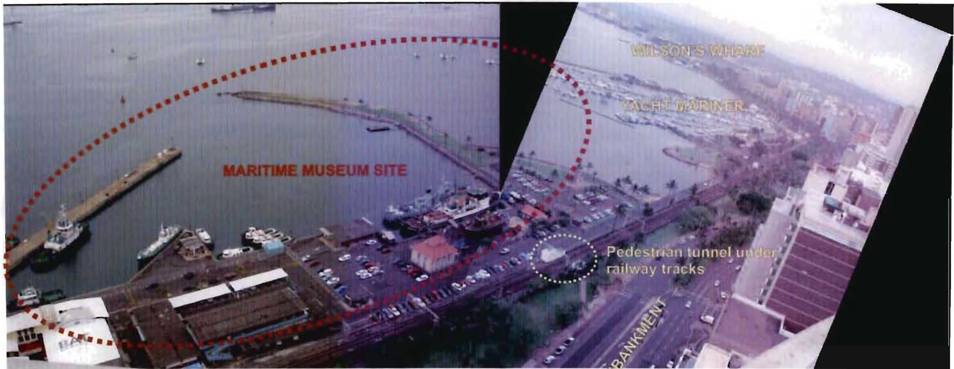
Figure 7.3_Aerial photograph of Maritime Museum site showing the existing conditions of the area.
