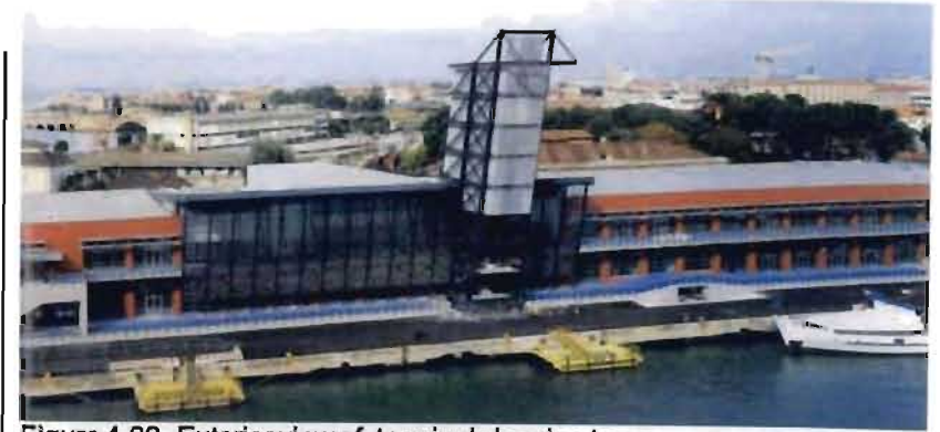
Figure 4.22_ Exterior view of terminal showing tower. (Dalco. 2003: 23)
