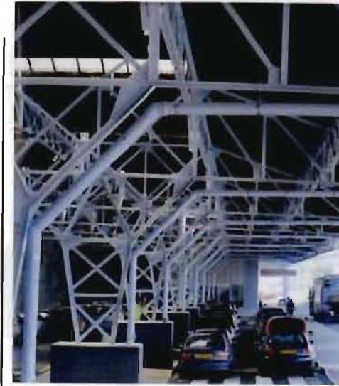
Figure 4.29_View of covered pick-up and drop-off area. (Baillui. 2003: 39)
