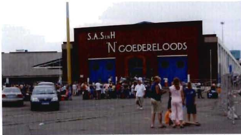
Figure 5.23_ Exterior photo showing main entrance on the north side of the terminal.
