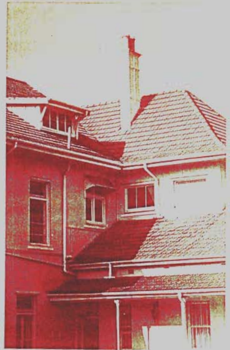
Junction between main house and service wing
