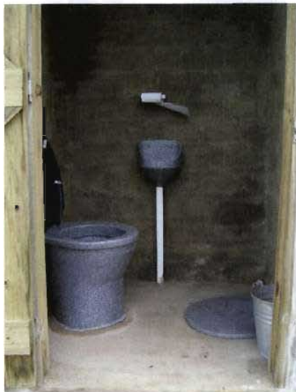
Plate 1: Inside view of the UD Toilet
