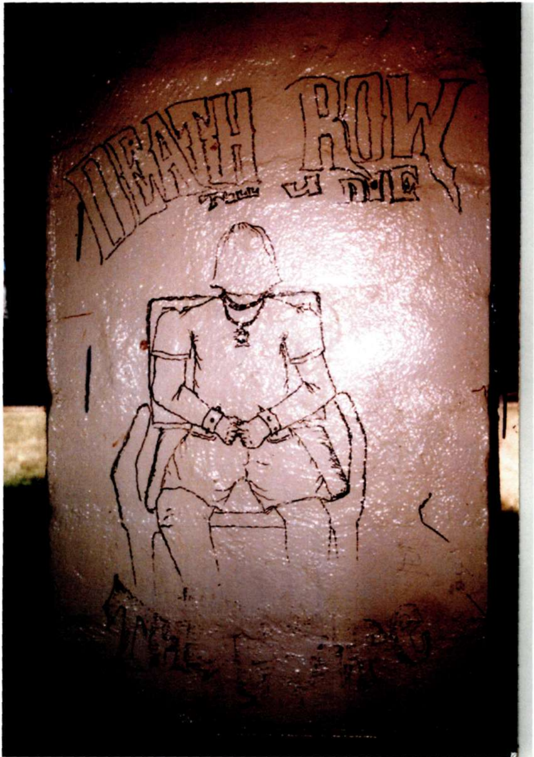
Picture 5: Graffiti in an Umzamo high school external wall
