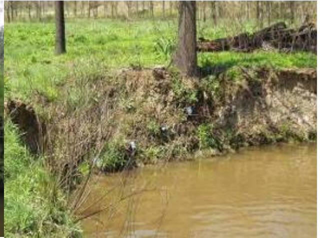
Survey 2003, Mpfana pipeline outfall (M2) post 3.2 m 3 /s discharge on the 02-10-03.
