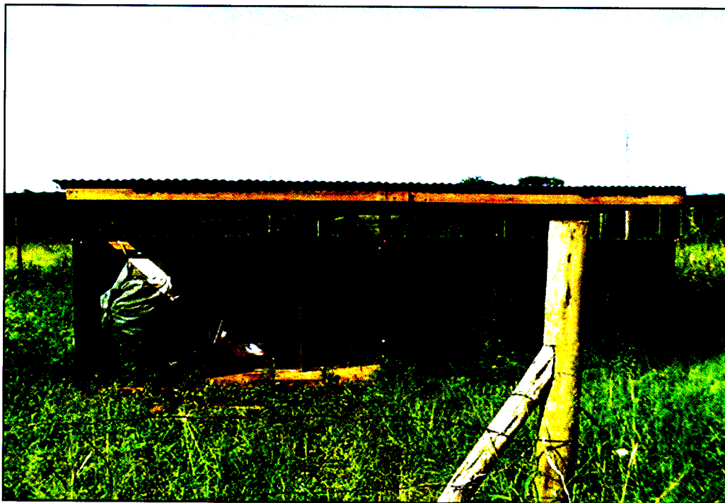
Figure 5.5 Waste shed, with waste collection trolley in the foreground
