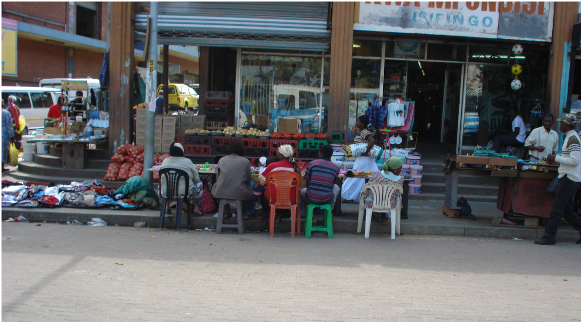
Photograph 8: Lack of pavement / road space management in terms of informal activities
