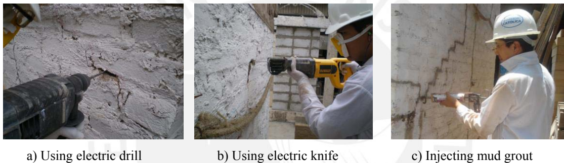
Figure 5. Opening seismic cracks and injecting mud grout.
