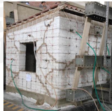
d) Repaired and strengthened model
