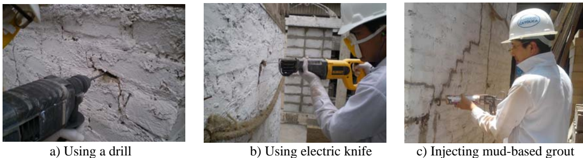
Figure 5. Opening and injecting the seismic cracks.
