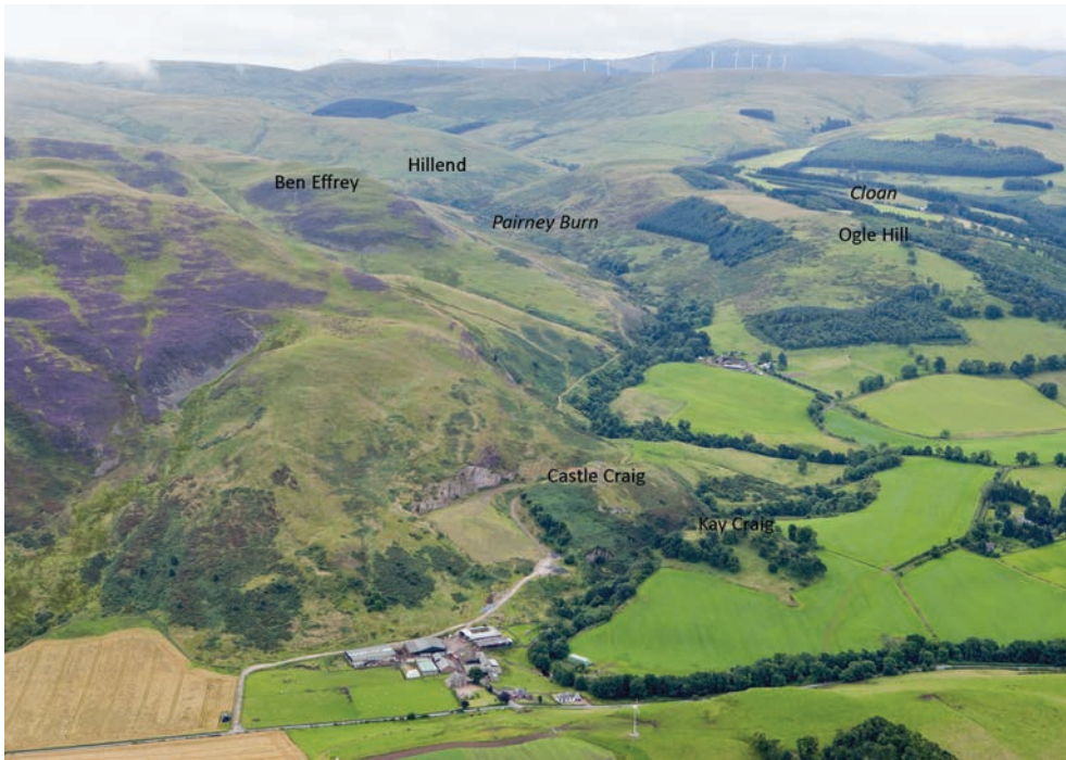
ILLUS 9 Aerial photograph looking south: hillforts of Ben Effrey, Castle Craig, Kay Craig and Ogle Hill; 18th-century farmstead Hillend; and Pairney Burn and Cloan (SERF)
