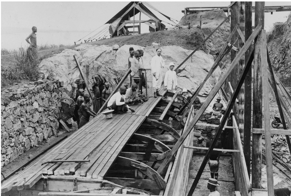
Figure 4. “Construction of the fort of Shinkakasa. Formwork of gallery I-II.” 1899. Photo: Mahieu. RMCA.
