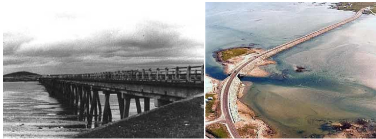
Figure 3. Single-lane concrete deck bridge (left) replaced by double-lane causeway (right) with a 15 metre span bridge
