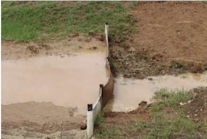
Figure 5-5: Silt traps placed on slopes or across small gullies to trap silt and slow water run-off rate.
