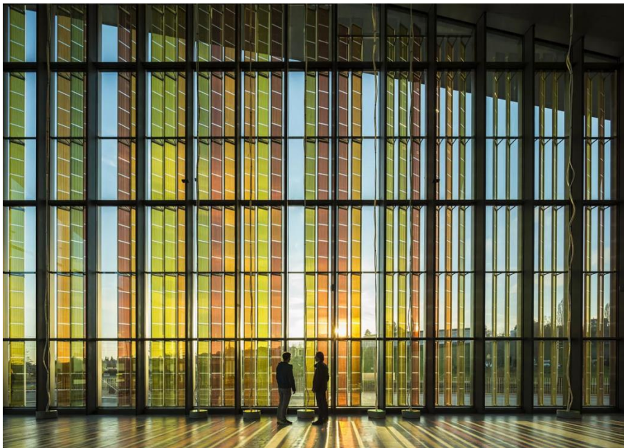
Figure 1.4. Glass façade composed by 300 m 2 of dye-sensitized solar cells demonstration modules in EPFL’s SwissTech Convention Center, Lausanne, Switzerland (adapted from 13 ).
