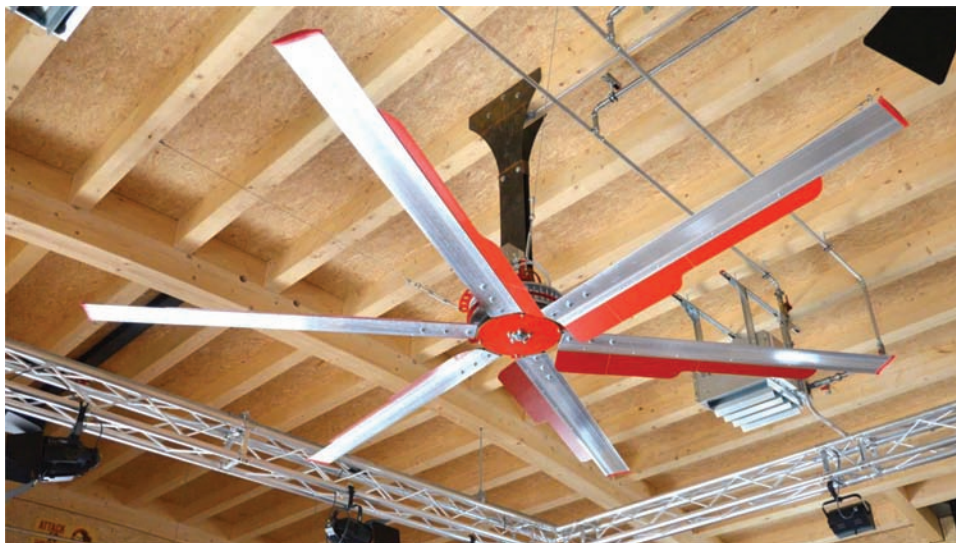
Figure 7. Ceiling fan for the control of the temperature in barns. The fan is fitted with five or six aluminum blades. The diameter of the fan varies from 3 to 5 m depending on the size of the barn.
