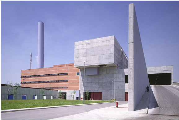
Fig. 12 Waste-to-energy tele-heating system Silla 2 in Milan (from http://www.a2a.it )
