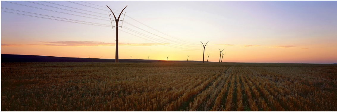
Fig. 28 Germogli pylon. HDA: Pylon Designer. Client: Terna. Competition Team: Hda, Rosenthal. Contractor: Tecnopali. Hda Team: Maria Angela Corsi (Competition Project Leader), Carla Zaccheddu, Francesco Cingolani, Pier Luigi Bucci, Gaëtan Kohler. Date: 2009–2013 (from http://www.hda-paris.com )
