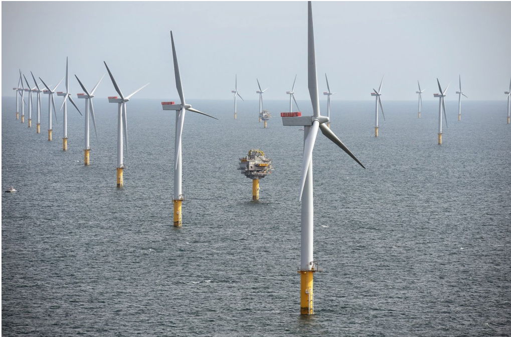
Fig. 26 Off shore wind turbines, Thanet Wind Farm, Thanet District (Kent), UK (from http://www.theguardian.com )
