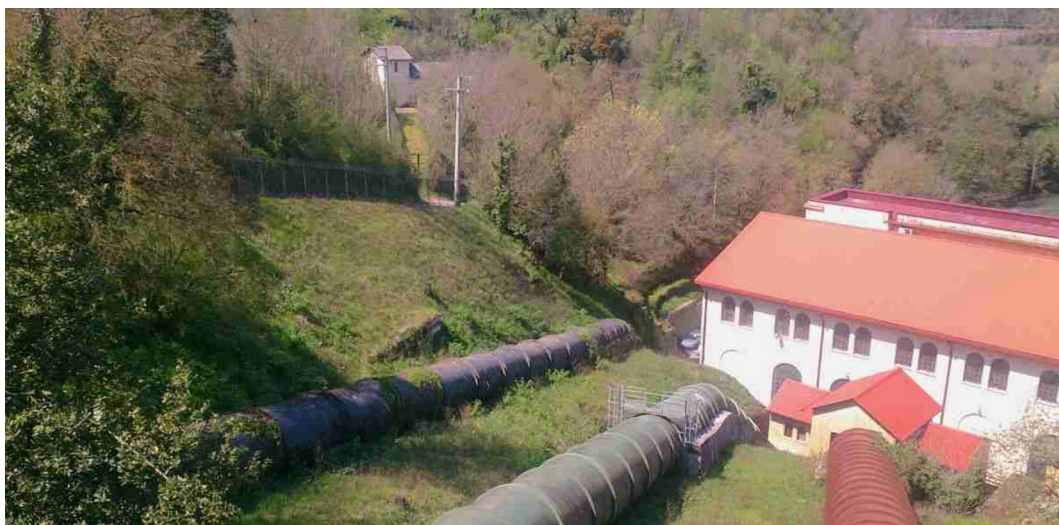
Fig. 18 Hydroelectric plant in Castel Madama IT (from www.atbrc.com )
