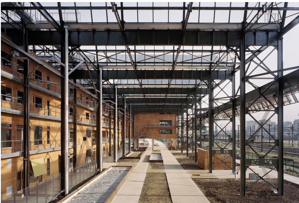
Fig. 27 Requalification of abandoned warehouse Halle Pajol in Paris with the inclusion of multiple public and private functions: the photovoltaic roof shelters also open spaces for orchards and common areas (from http://www.jourda-architectes.com )
