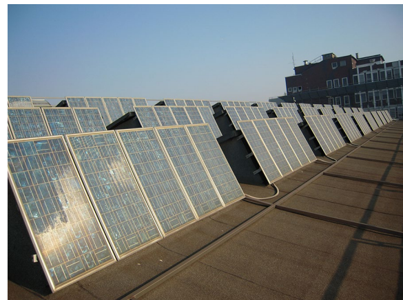
Fig. 11 Photovoltaic plant of medium size (Library roof plant of Politecnico of Milano. Picture by authors)
