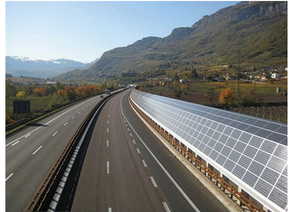
Fig. 15 Photovoltaic railing and guardrails photovoltaic parkings. (Here the Brennero highway in Italy from http://www.autobrennero.it )
