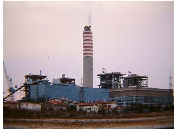
Fig. 22 Thermoelectric plant in Monfalcone, IT (from http://www.a2a.it )
