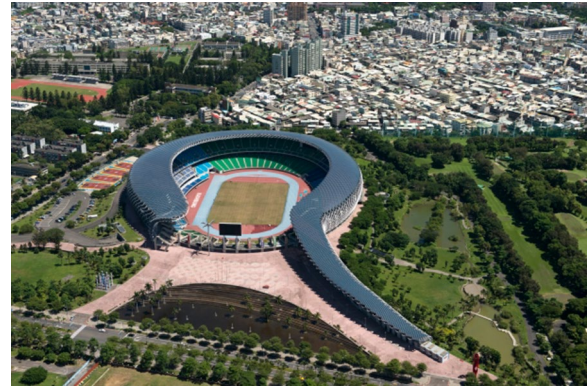
Fig. 19 Kaoshiung stadium, T. Ito, 2009, Kaoshiung, Taiwan (from https://k720.kcg.gov.tw )
