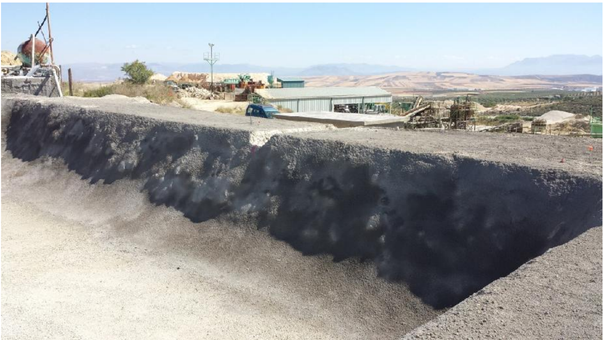
Figure 59. Canal to connect solar pond with auxiliary pond 2
