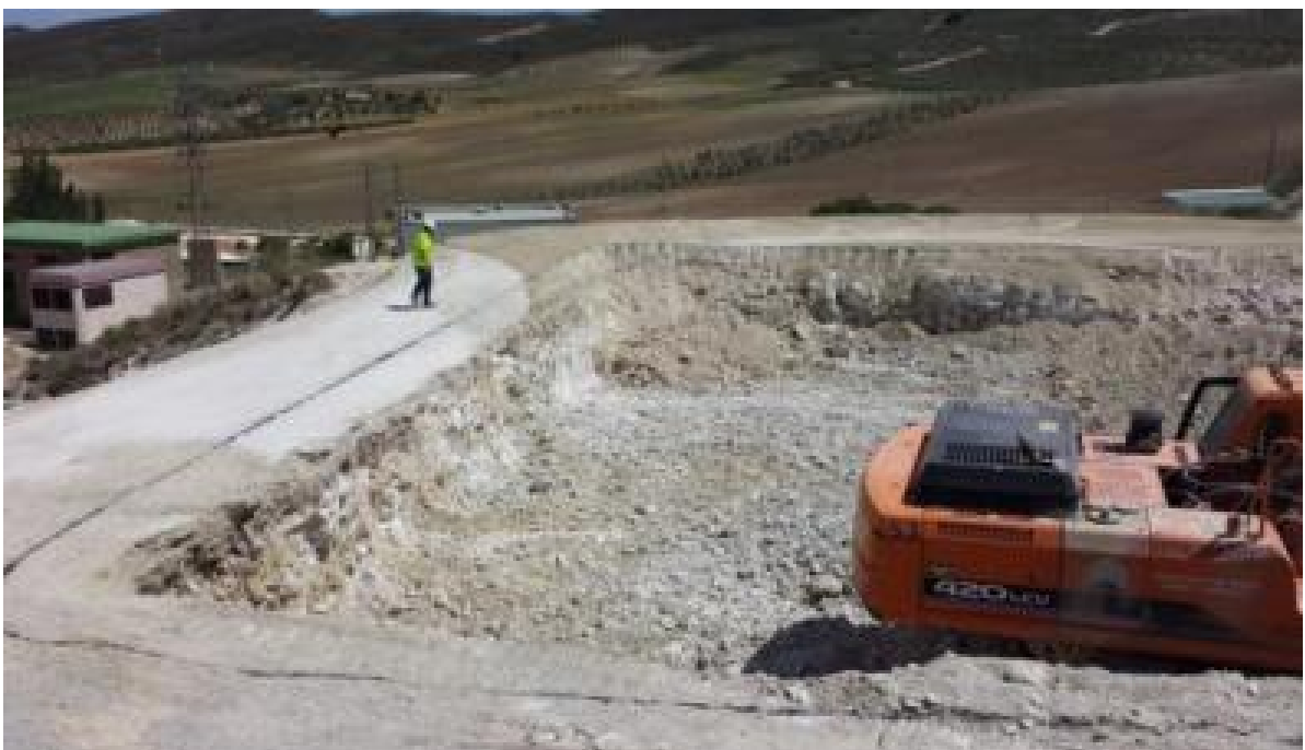
Figure 52. First phase of the excavation process
