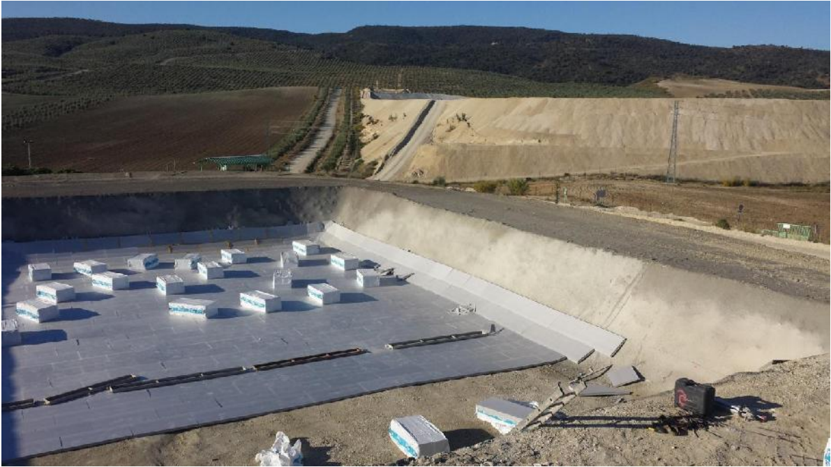
Figure 63. Start of the thermal insulation installation process
