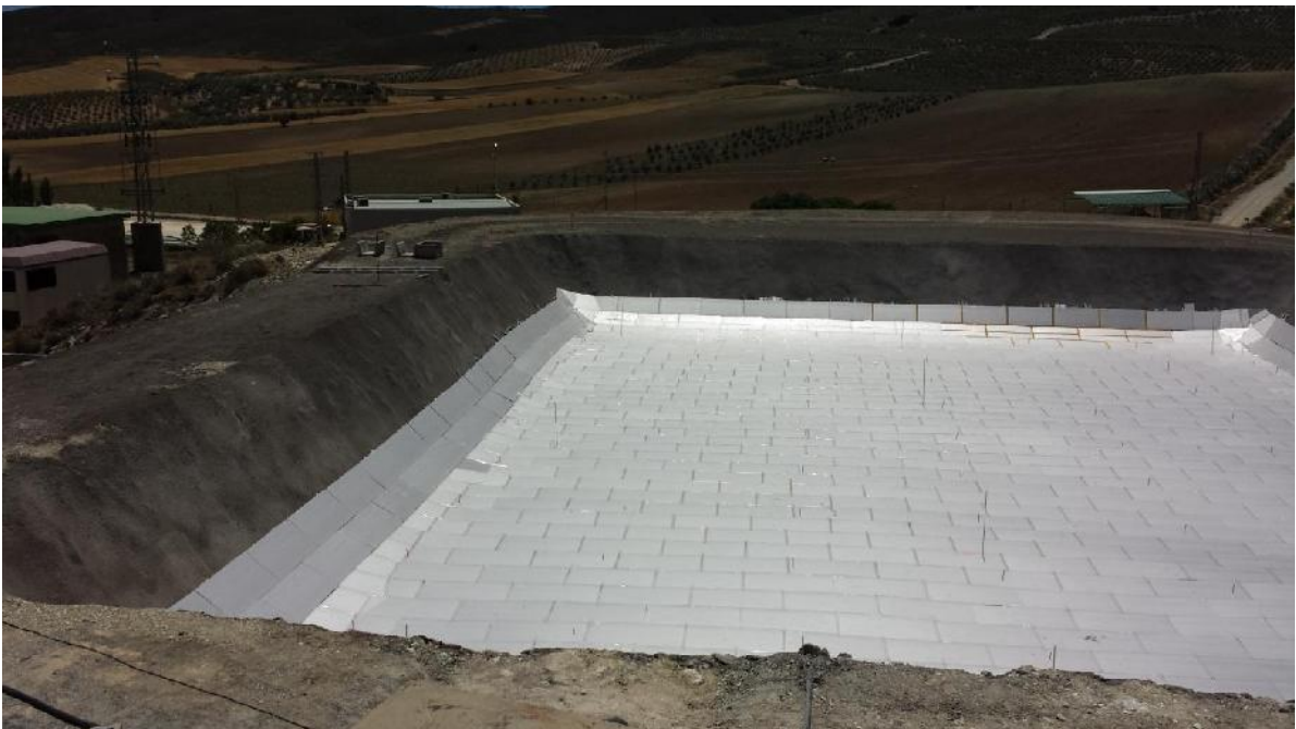
Figure 64. End of the process of placing the first layer of insulation
