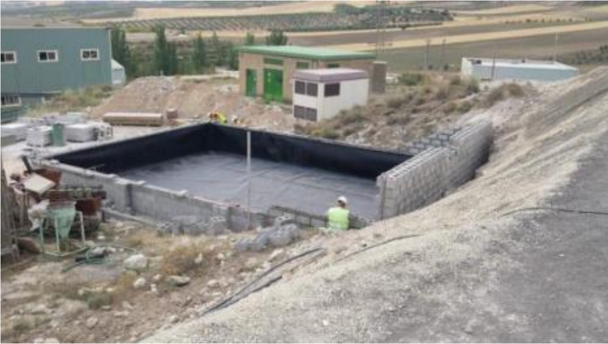
Figure 89. Laying the layer second layer of PVC
