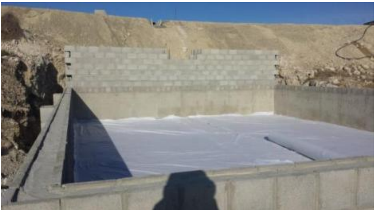
Figure 88. Laying the geotextile layer
