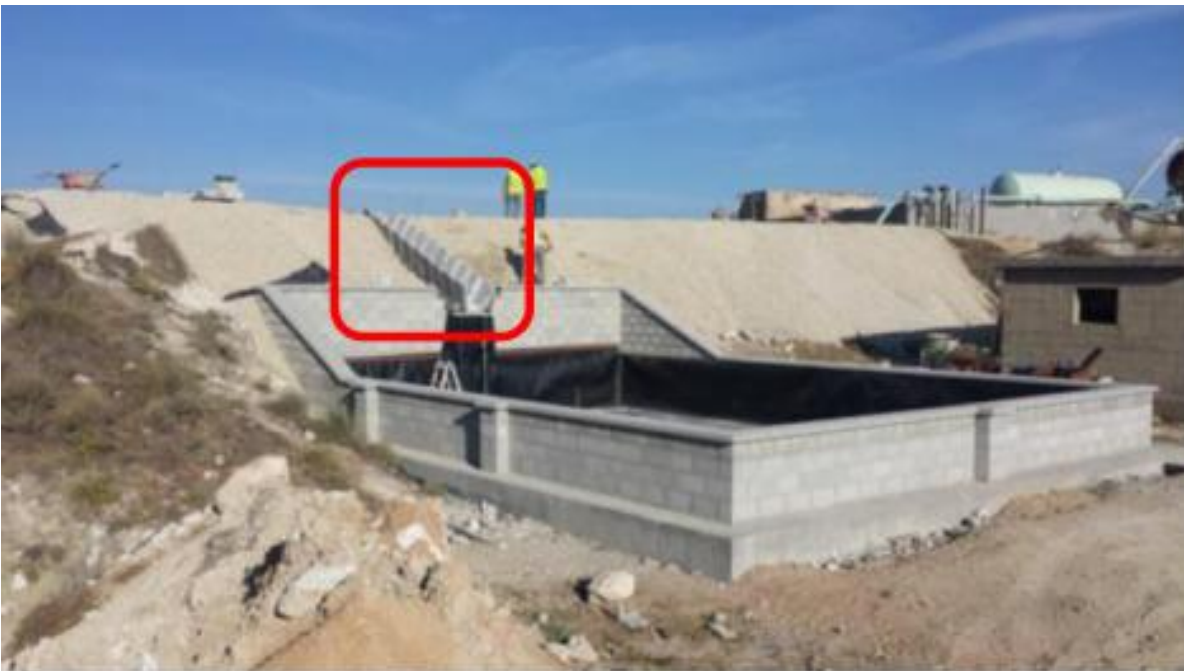
Figure 90. Final aspect of the auxiliary pond and union with the solar pond (red)
