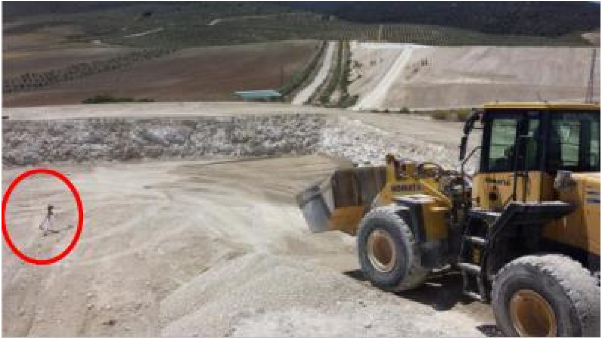
Figure 55. Land leveling on the base of the pond
