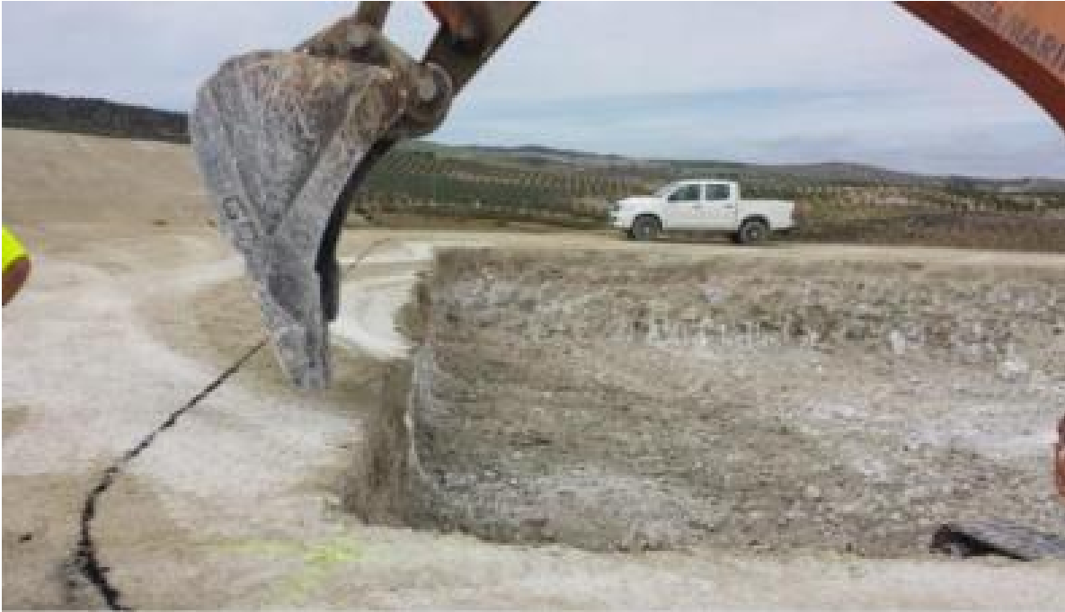
Figure 53. Second phase the excavation process
