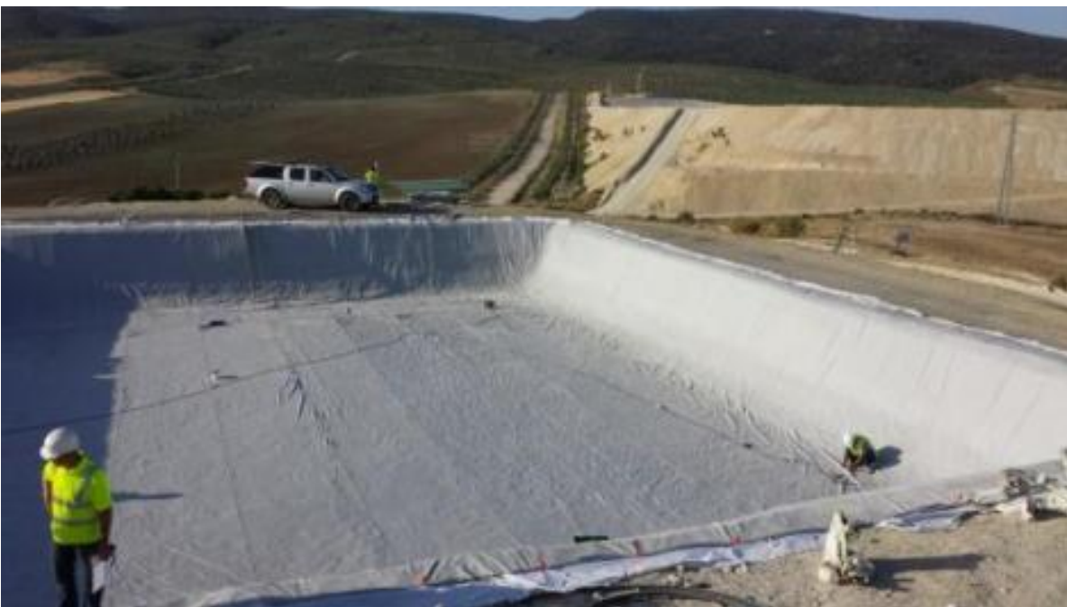
Figure 70. End of the process of placing the third layer of insulation
