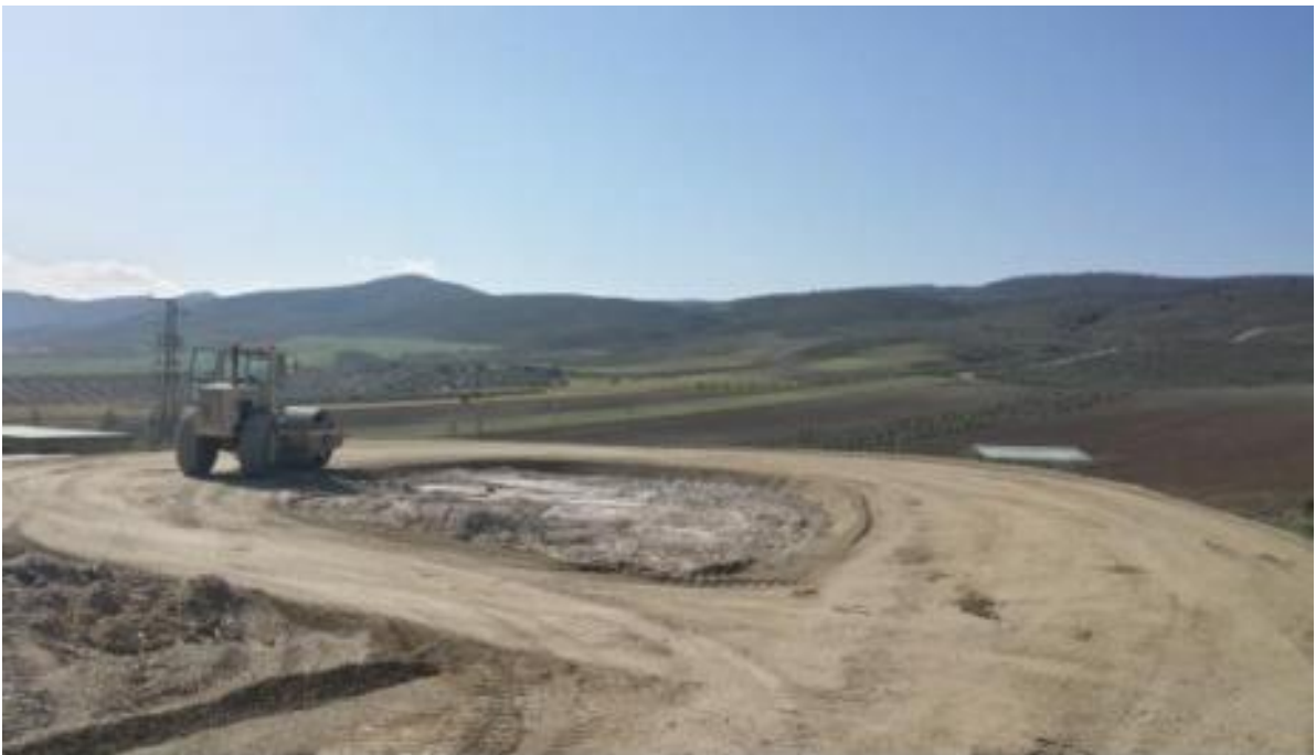
Figure 49. Compaction of the ground
