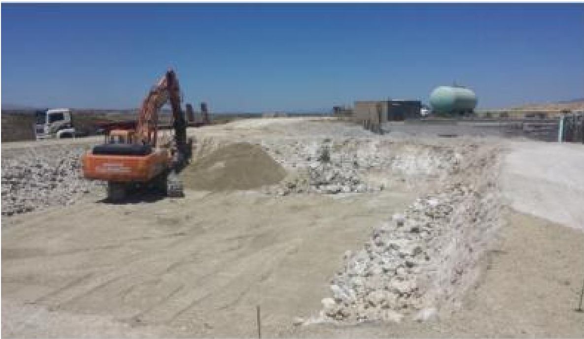
Figure 54. End of the excavation process
