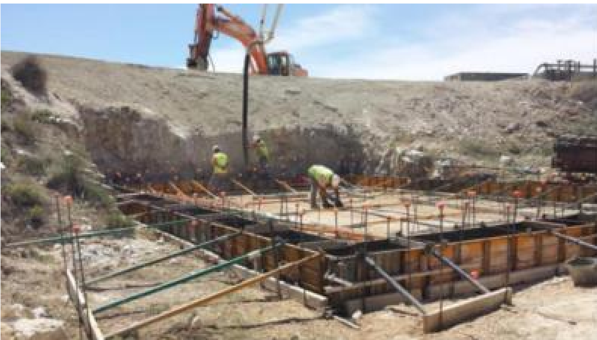
Figure 86. Structure of the auxiliary pond
