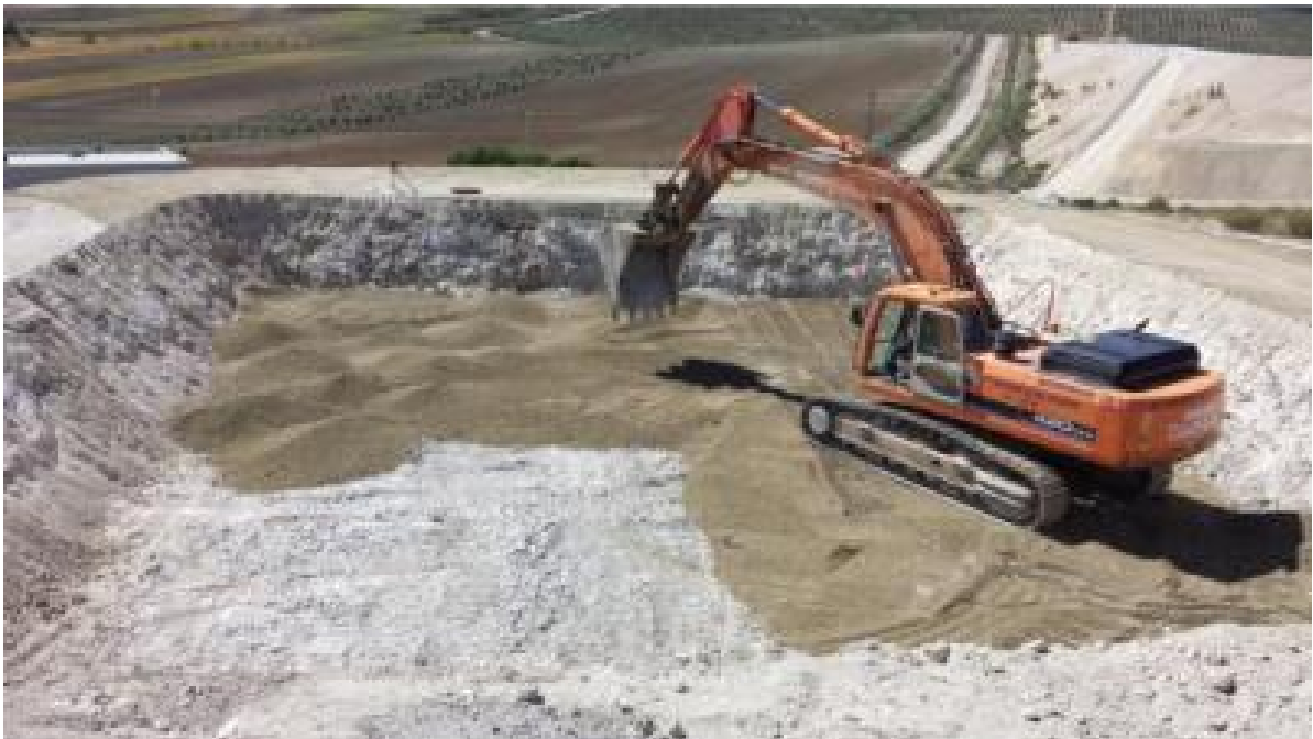
Figure 56. Addition of material on the walls of the pond
