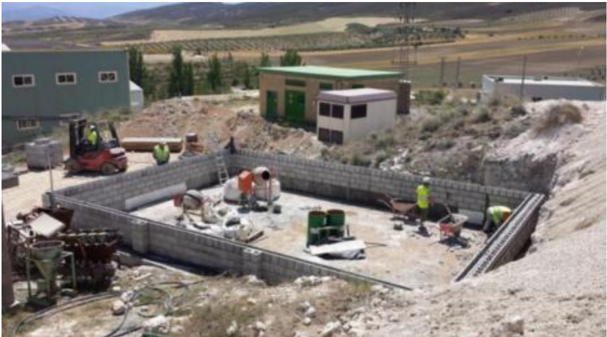
Figure 87. Construction of the walls of the auxiliary pond
