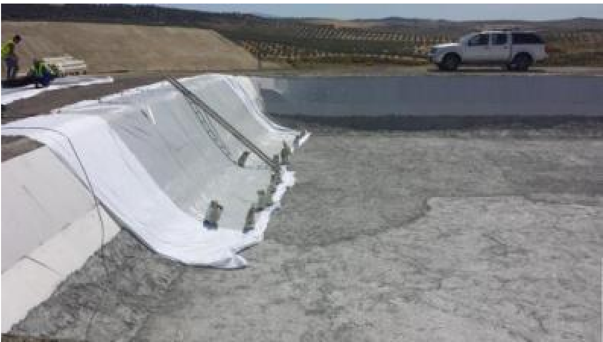
Figure 68. Laying the geotextile layer
