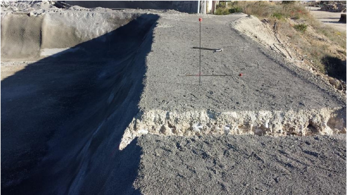
Figure 58. Canal to connect solar pond with auxiliary pond 1
