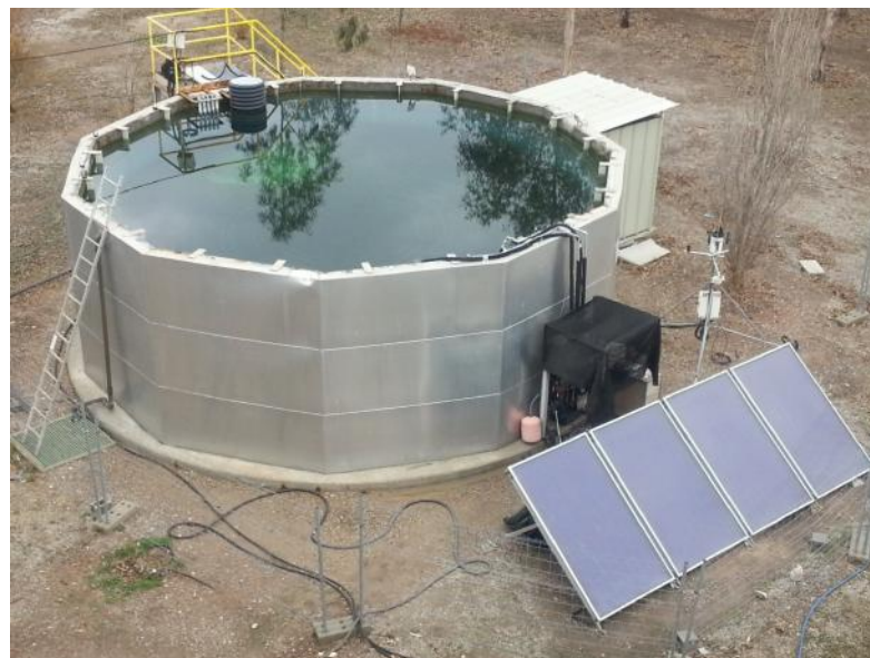
Figure 12. Solar pond Martorell
