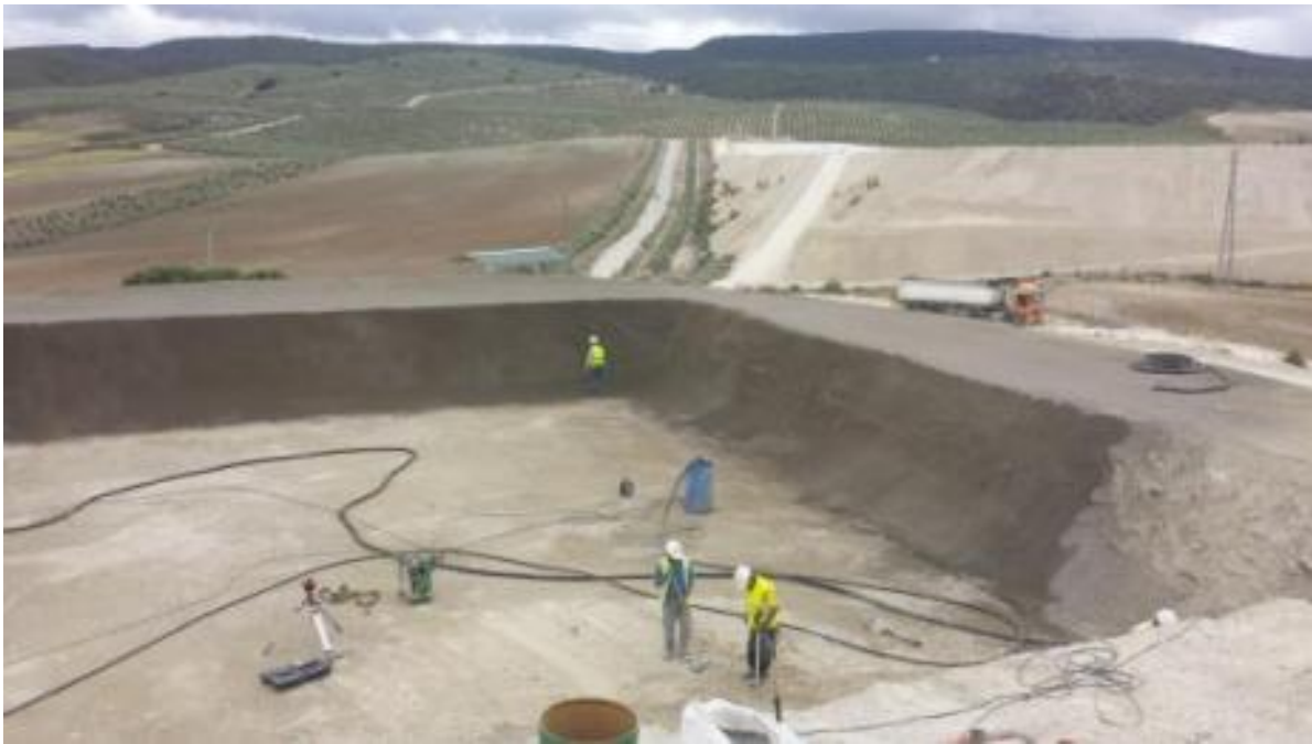
Figure 61. Concrete layer on the walls to waterproof the system
