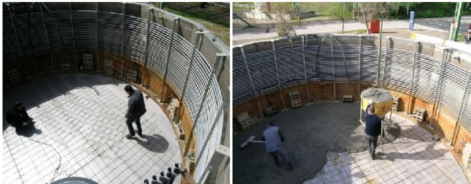
Figure 14. Insulation and concrete process installation in solar pond Martorell
