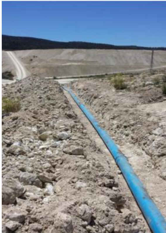
Figure 46. New location of the freshwater pipe
