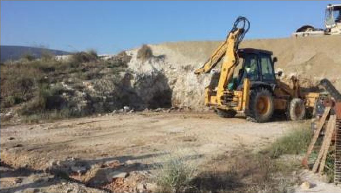
Figure 85. Preparation of the ground of the auxiliary pond
