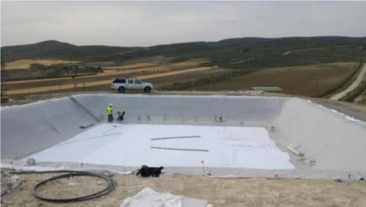
Figure 69. Placement of PVC on the geotextile layer
