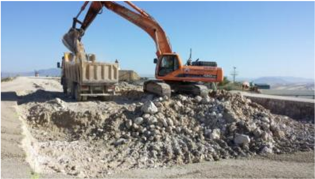
Figure 51. Start of excavation process
