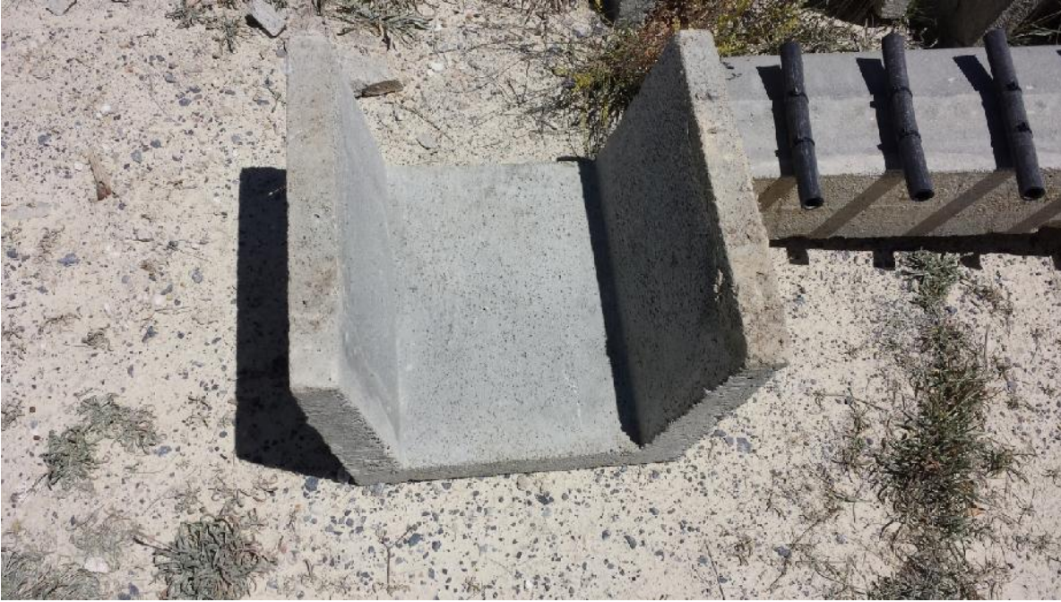
Figure 60. Concrete piece used in construction of the overflow system
