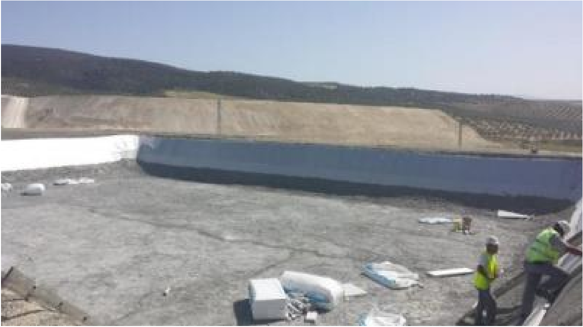
Figure 67. End of the process of placing the second layer of insulation
