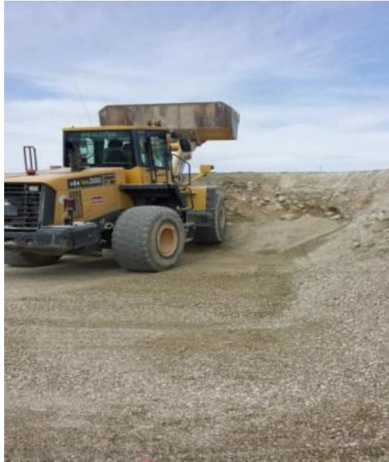
Figure 57. Addition of material on the base of the pond
