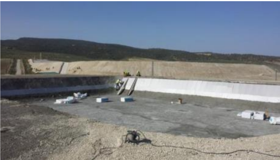
Figure 66. Laying the ChovAFOAM material on the walls.
