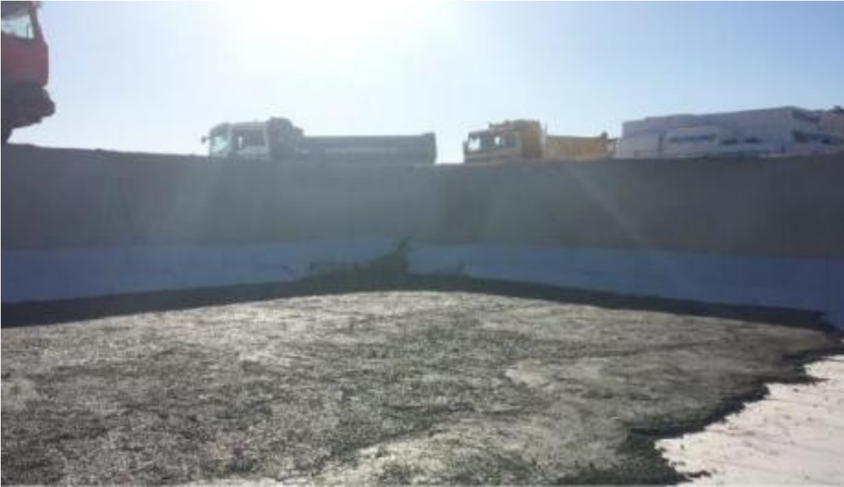
Figure 65. Laying the extended clay layer
