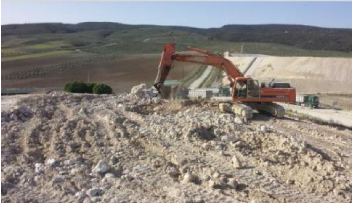
Figure 48. Removal of rock
