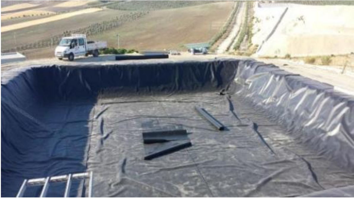
Figure 71. End of the process of placing the quarter layer of insulation
