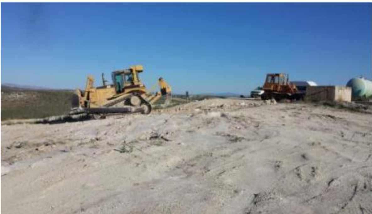
Figure 47. Preparation of the ground
