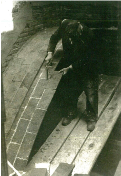
Fig. 1. Construction “in space” of a tile-vaulted stair [10].
