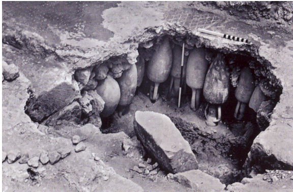
Figure 3: Amphorae laid vertically and covered with compacted infill material acting as a form of a static air cavity (Rabat Malta).
