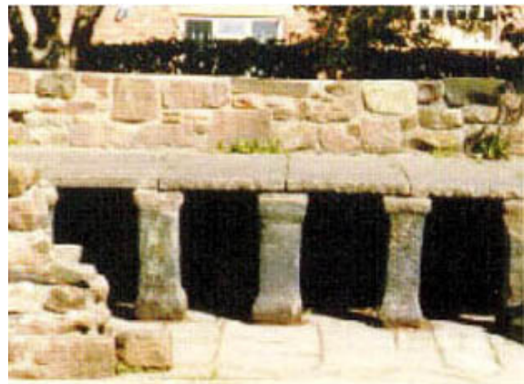
Figure 1: raised floor on stump walls with gaping openings for cross-ventilation
