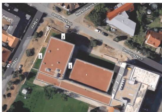
Figure 11. Measuring points outside the building (Source: https://www.google.com/maps/place/Debrecen ).
