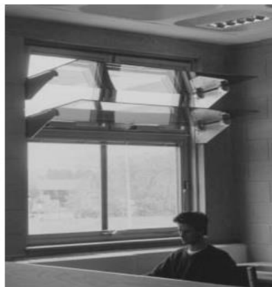
Figure 1.4: Le système light shelf (Source: Ruck et al., 2000)
