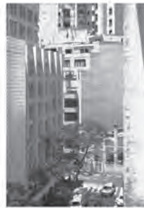
11. PAINTED FLANK WALLS PRESENT STRONG ATTRACTIVE SILHOUETTE
