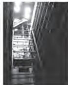
37. BASEMENT CAR PARK ACCESS PRESENTS UNEXPECTED CUTS INTO GROUND. 38. MECHANICAL CAR PARK OFFERS WIDE INTERIOR ATHLUM.
