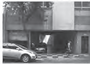
13. LIGHT SHAFT CONTRAST-DARK UNDERCROFT
