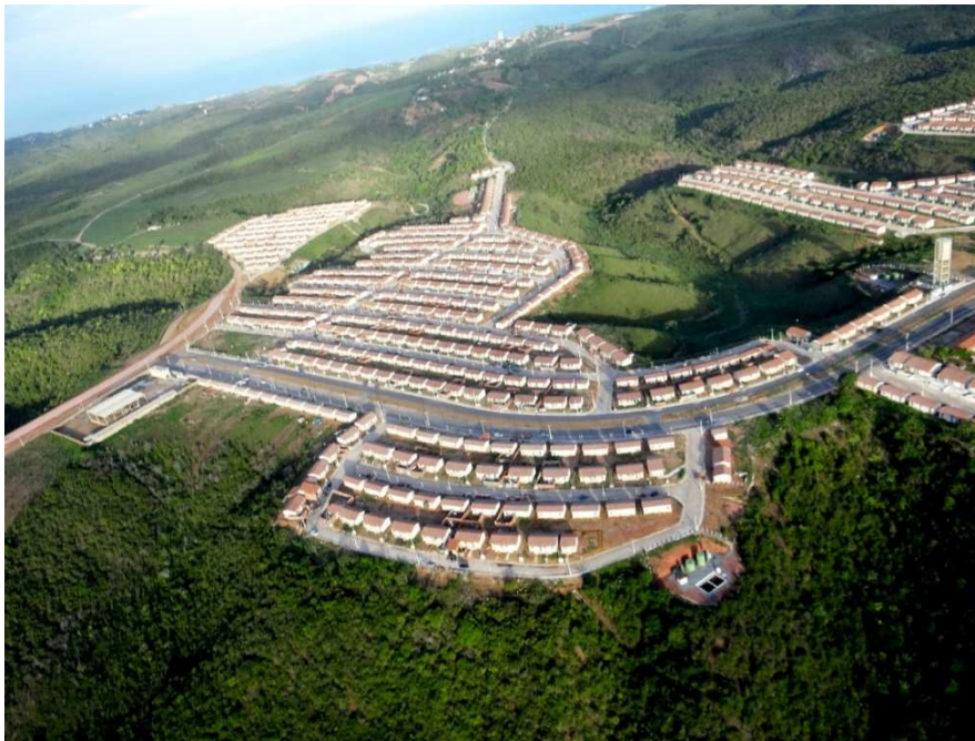
Figure 3: Maceió-AL, Minha Casa Minha Vida social housing aerial view, 2014. Photography courtesy of the Laboratory QUAPÁ, from the Faculty of Architecture and Urbanism, University of São Paulo – FAUUSP, Brazil.
