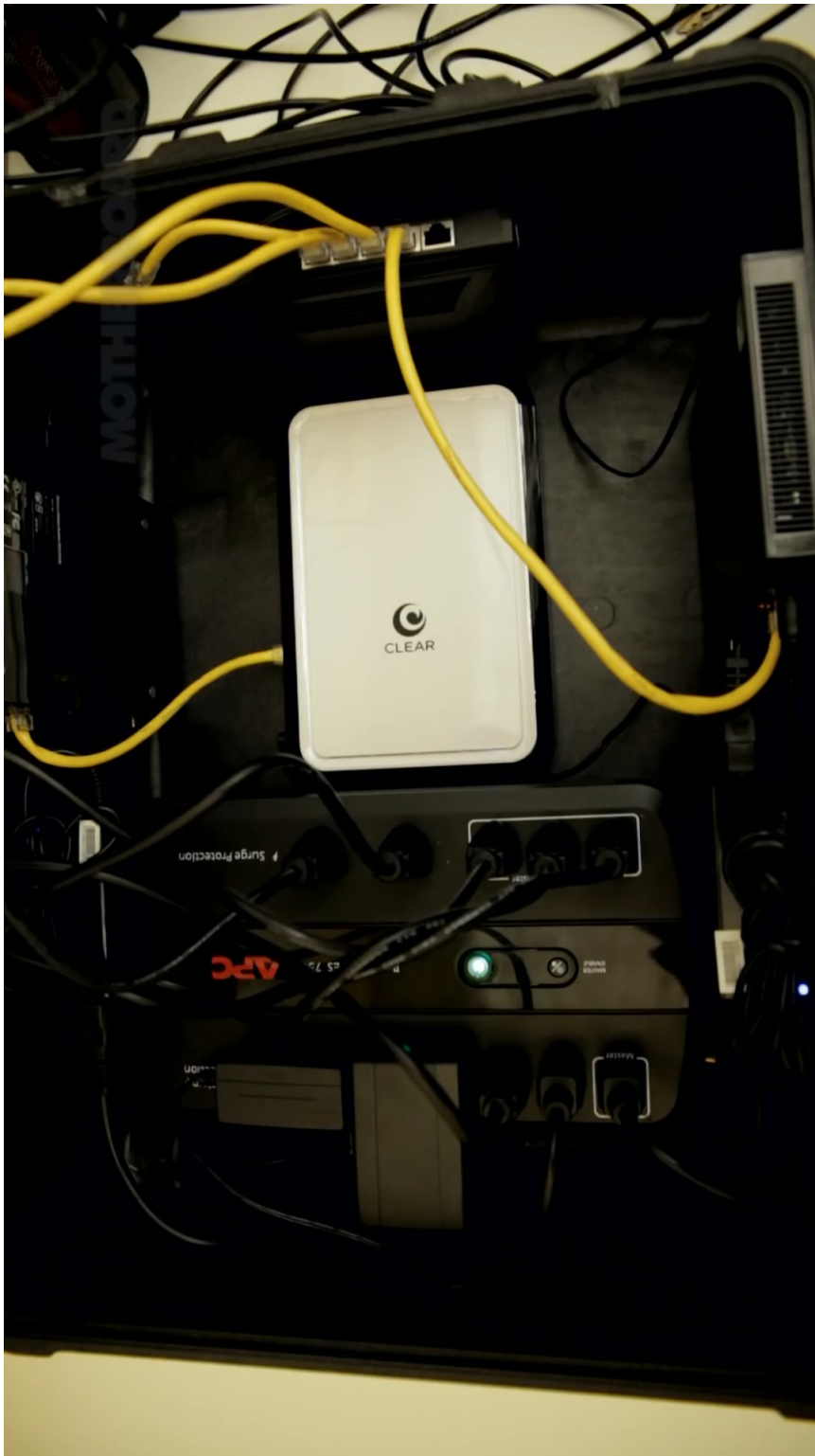
Figure 6: Freedom Tower enclosure (better view) (Motherboard 2012).
