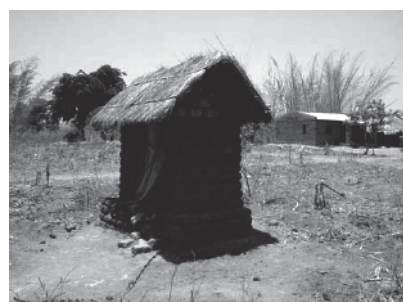
Figure 3 A typical traditional pit latrine in Malawi
