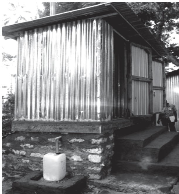
Figure 6b Skyloo with urine diversion into a plastic container
