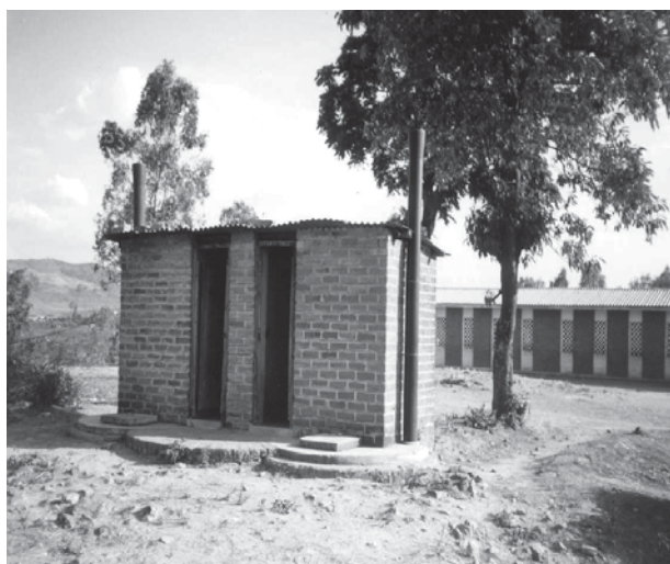
Photograph 2. Example of improved pit latrine
