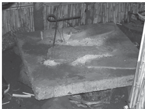
Plate 3b: A complete fully covered Eco-sanitation latrine.
