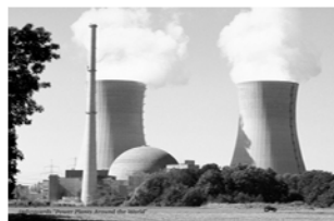
Nuclear Power Station
