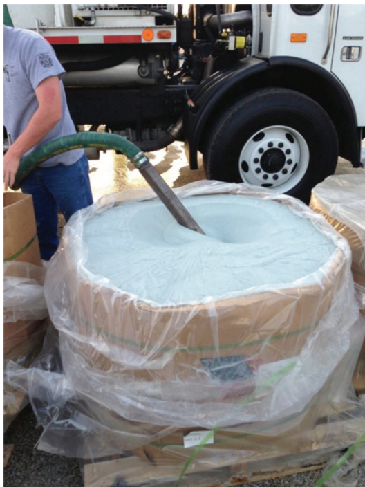
Figure 4.3 Sucking glass beads from pallet on ground into the bead tank.
