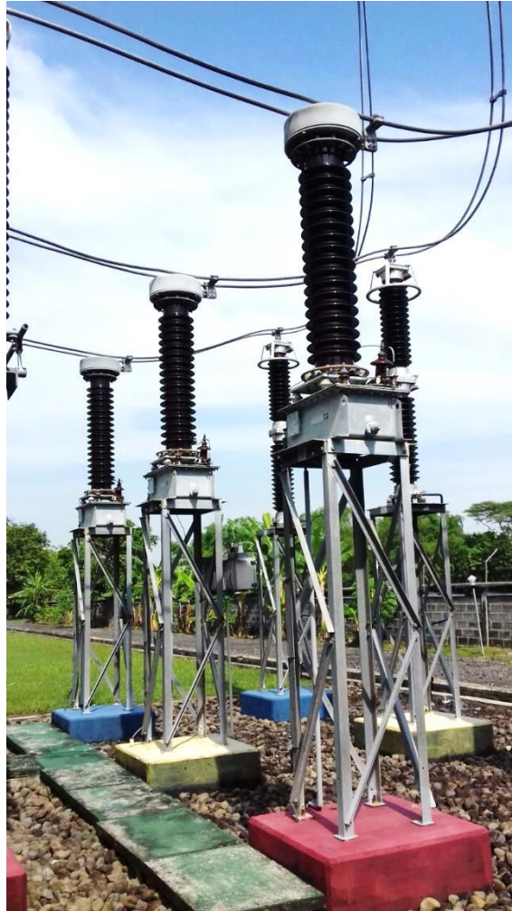
Gambar 8. Potential Transformator
