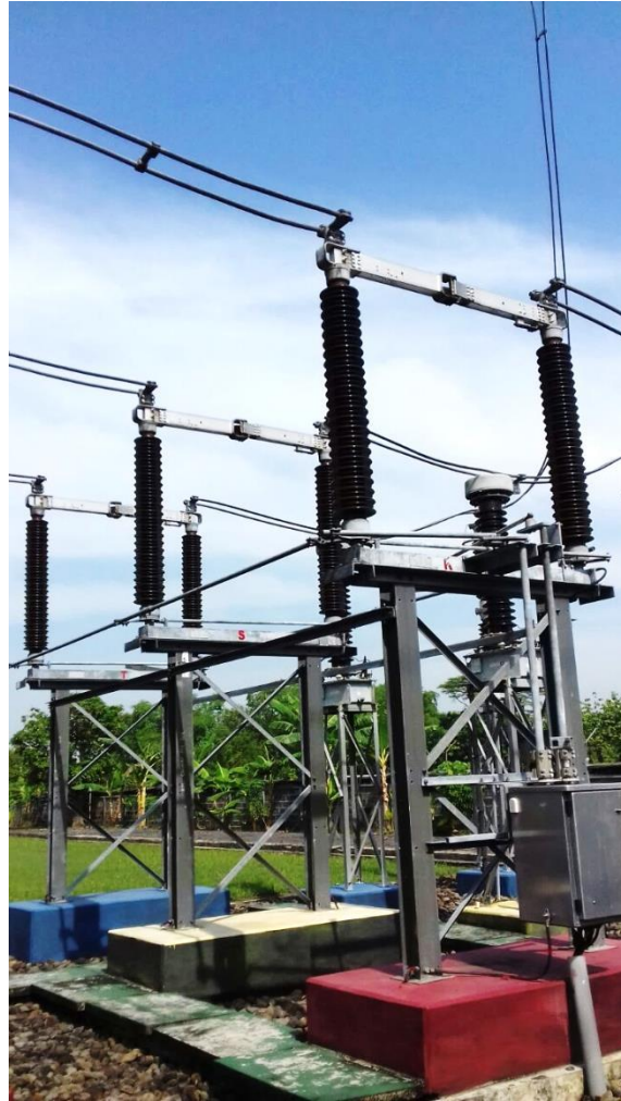
Gambar 5. Disconnecting Switch
