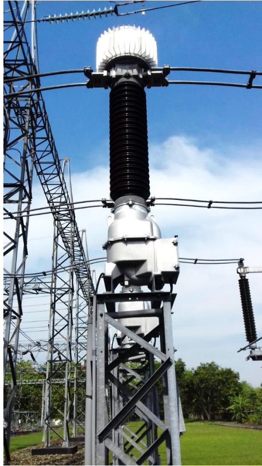
Gambar 7. Current Transformator
