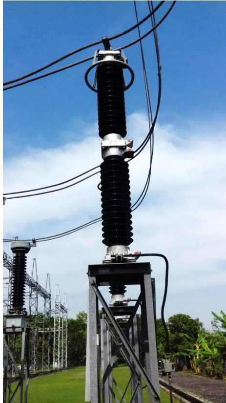
Gambar 6. Lightning Arrester
