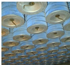
Figure 15: Cylindrical Cartridge Self-cleaning Filter. Source: Donaldson (GTS-102)
