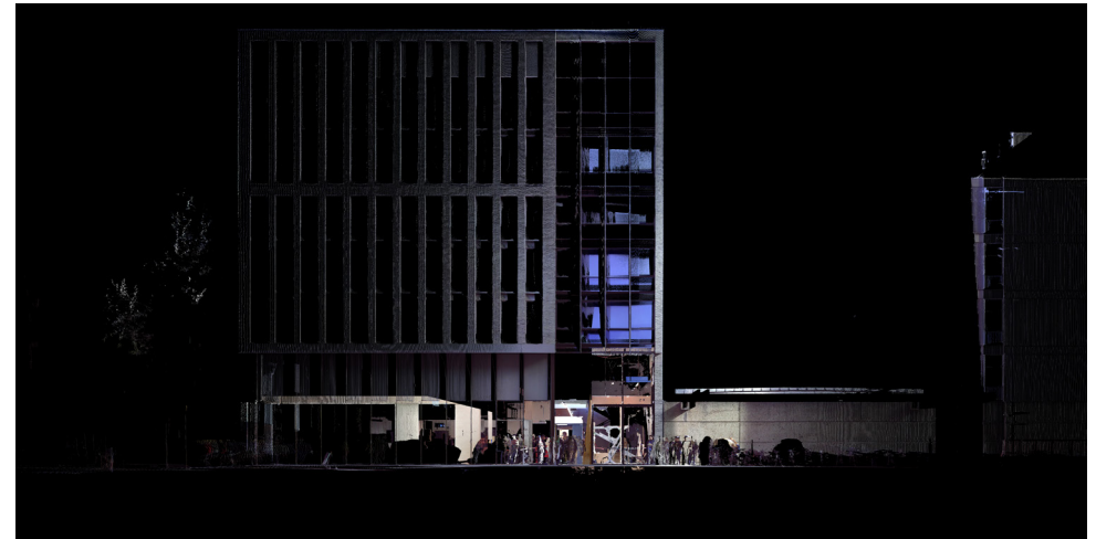
Figure 2. Elevation of the main façade of 22 Gordon Street. (Source: author).
