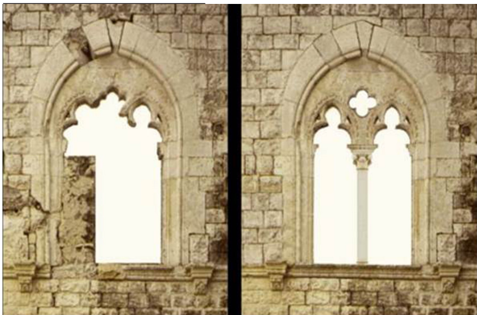
Figure 9. Virtual restoration of a two-lane window of S. Giovanni in castrum Church in Bisceglie. (Source: courtesy of CNR, ITC of Bari).
